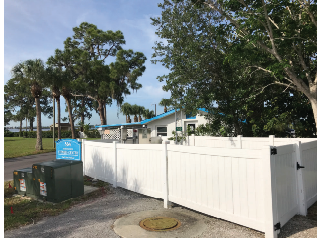
Figure 4: Overview of Lift Station No. 519 (Colony Cove 3)
