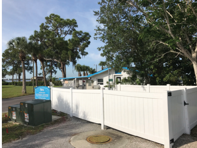
Figure 6: Overview of Lift Station No. 519 (Colony Cove 3)
