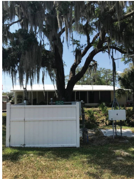
Figure 7: Overview of Lift Station No. 520 (Colony Cove 4)
