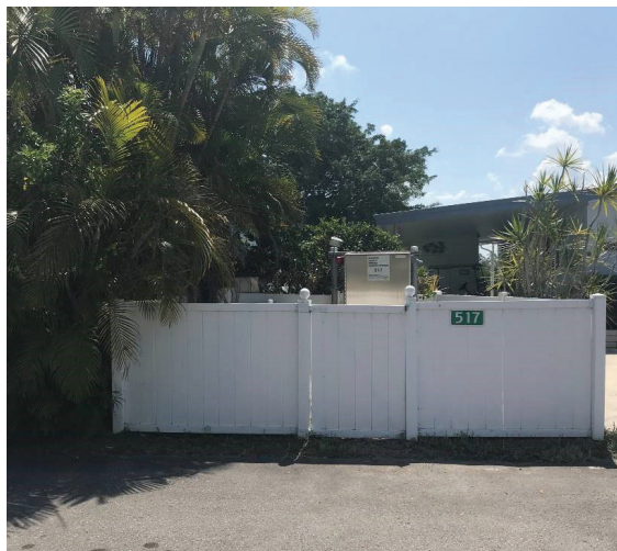
Figure 4: Overview of Lift Station No. 517 (Colony Cove 1)
