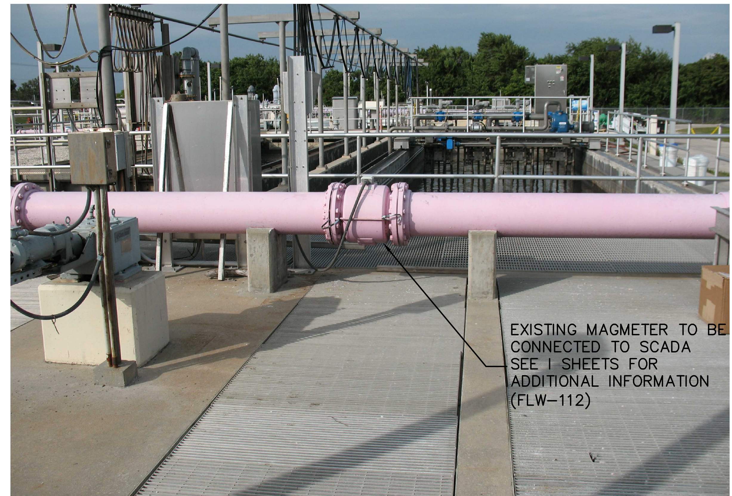
ABW FILTERS 1 & 2 METER ASSEMBLY
