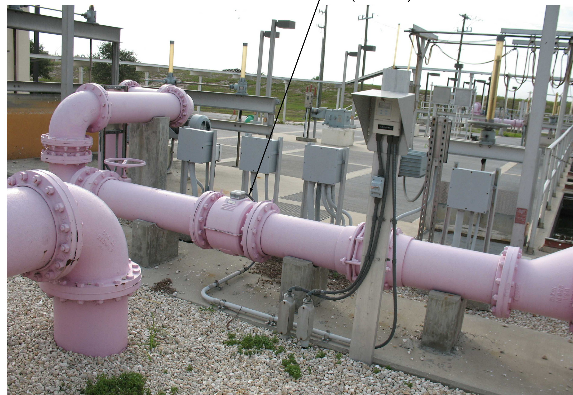
ABW FILTERS 3, 4 & 5 METER ASSEMBLY
