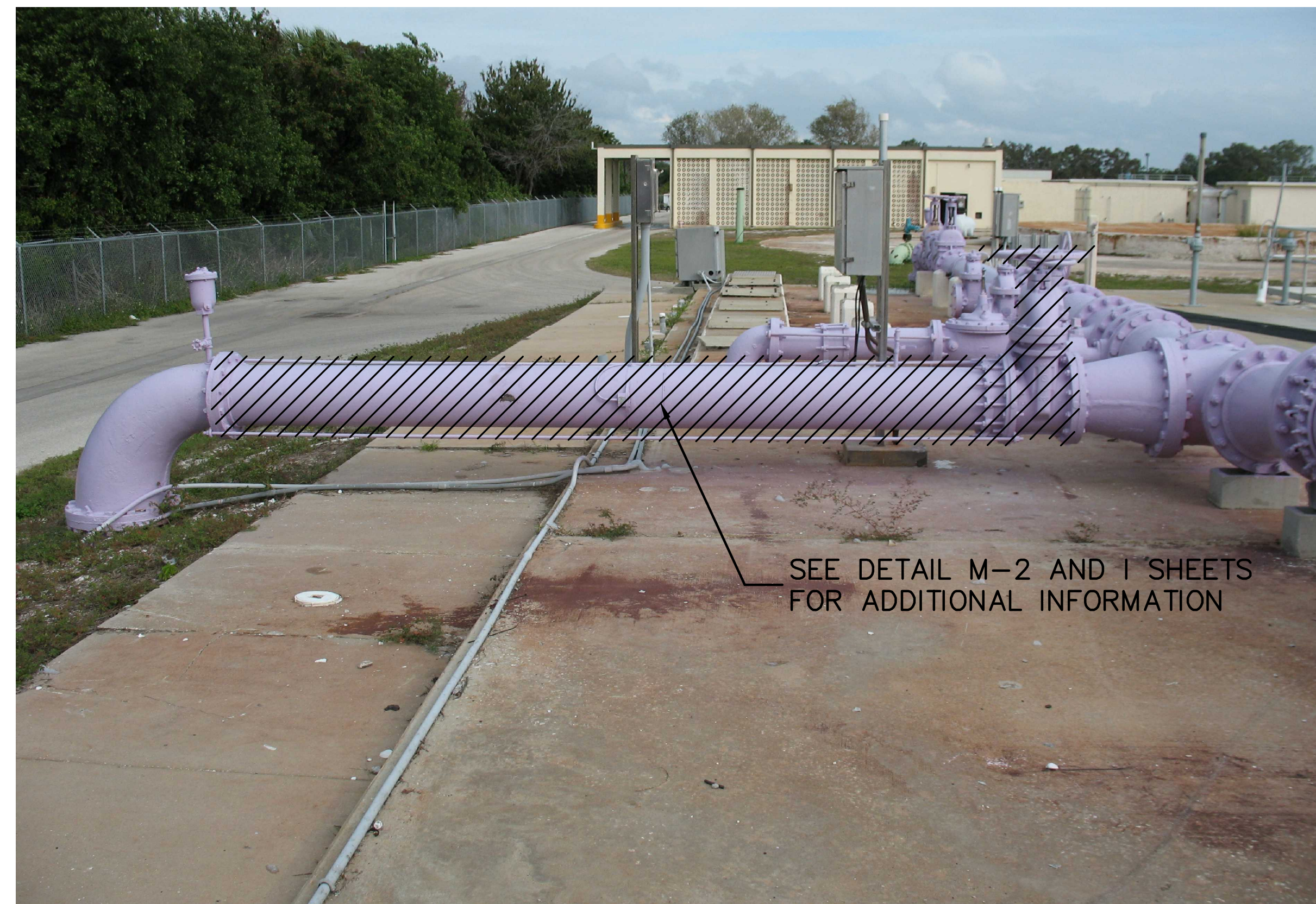
IRRIGATION METER ASSEMBLY DEMO
