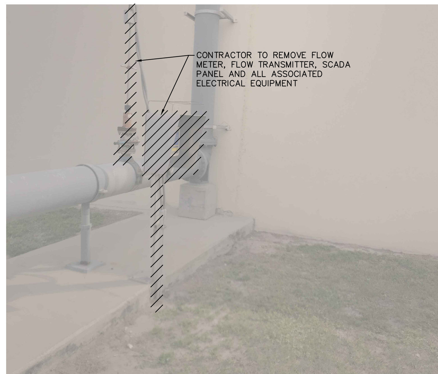
EX. NORTH AND SOUTH EQUALIZATION TANK LEACHATE FLOW METER DEMOLITION
