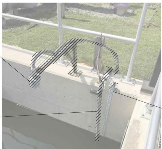
CUT STAFF GAUGE SO THAT TOP OF GAUGE IS FLUSH WITH FLOOR. REPLACE FLOOR MOUNT WITH WALL MOUNT BRACKET.
