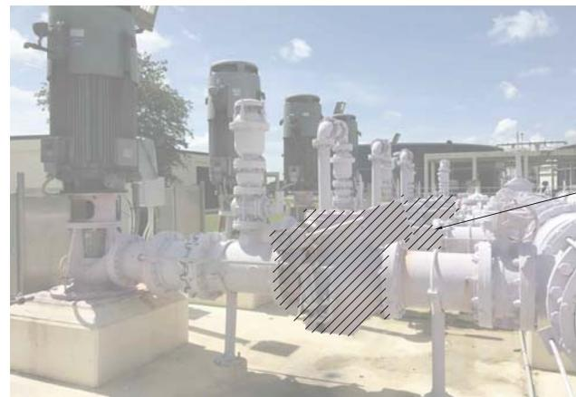
REMOVE AND REPLACE 12" CHECK VALVE (TYP. OF 4)
