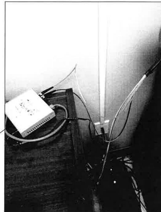
EXISTING FIBER OPTIC NETWORK SWITCH AND UPS
