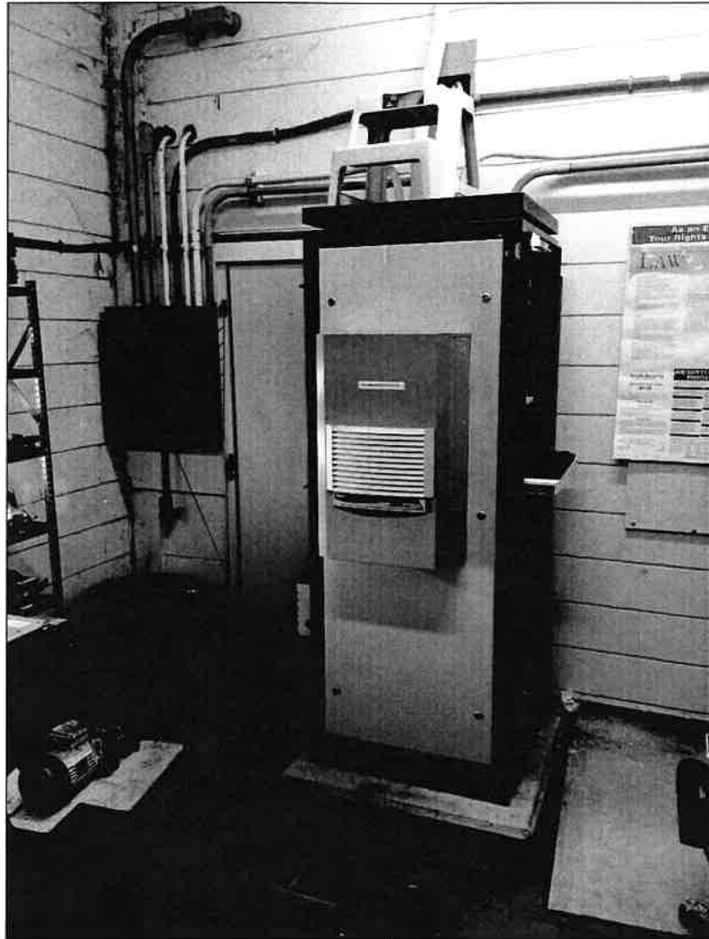
REPLACE EXISTING ANALOG TERMINATION CABINET FOR DCU-3
