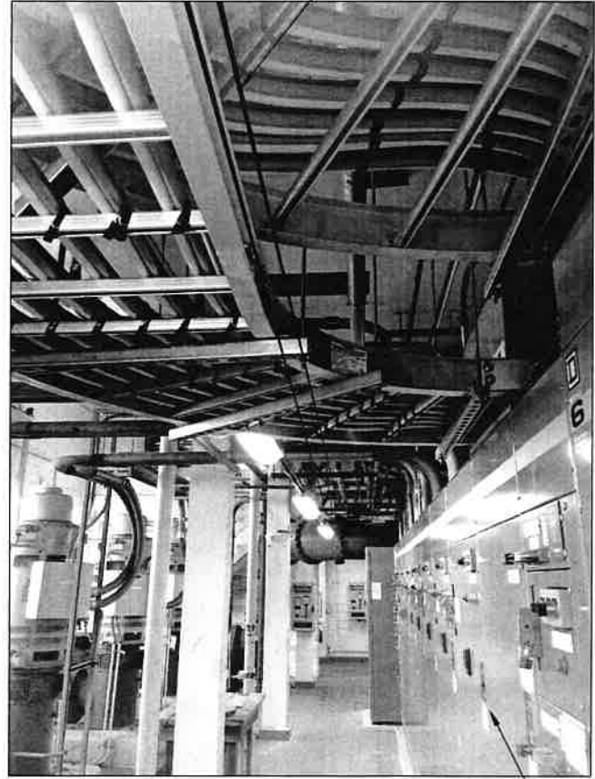
GROUND FLOOR LEVEL VIEWING WEST TOWARDS FILTER GALLERY
