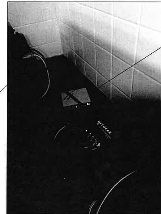
EXISTING FIBER OPTIC NETWORK SWITCH LOCATED BEHIND EXISTING SCADA WORKSTATION
