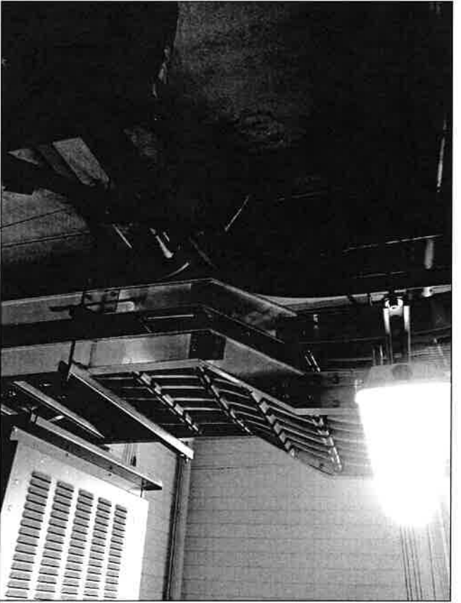
CONTROL ROOM FLOOR FROM GROUND LEVEL
