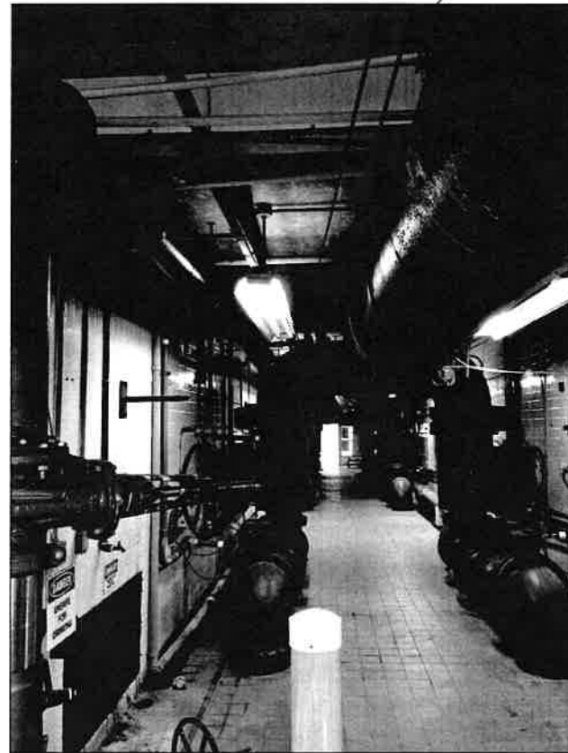
FILTER GALLERY A VIEWING NORTH TOWARDS FILTER GALLERY B
