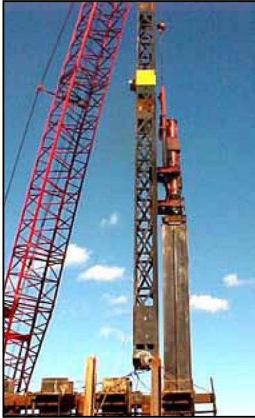
D62-42 in a stand-off driving Kingpile.
