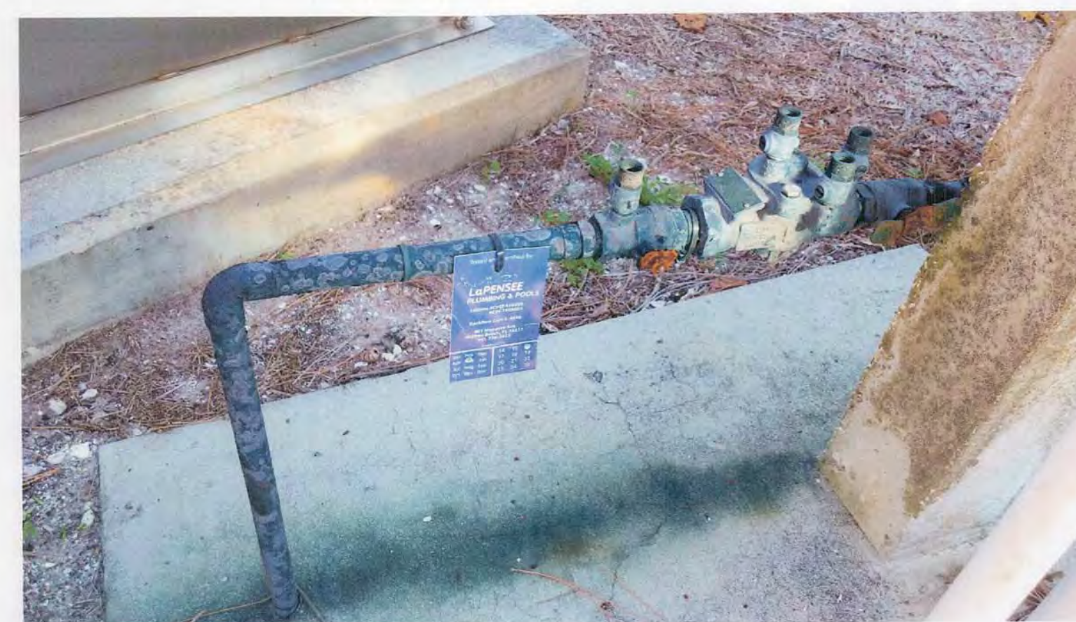
REPLACE 3/4-INCH REDUCED PRESSURE (RPZ) BFP AND SPIGOT
