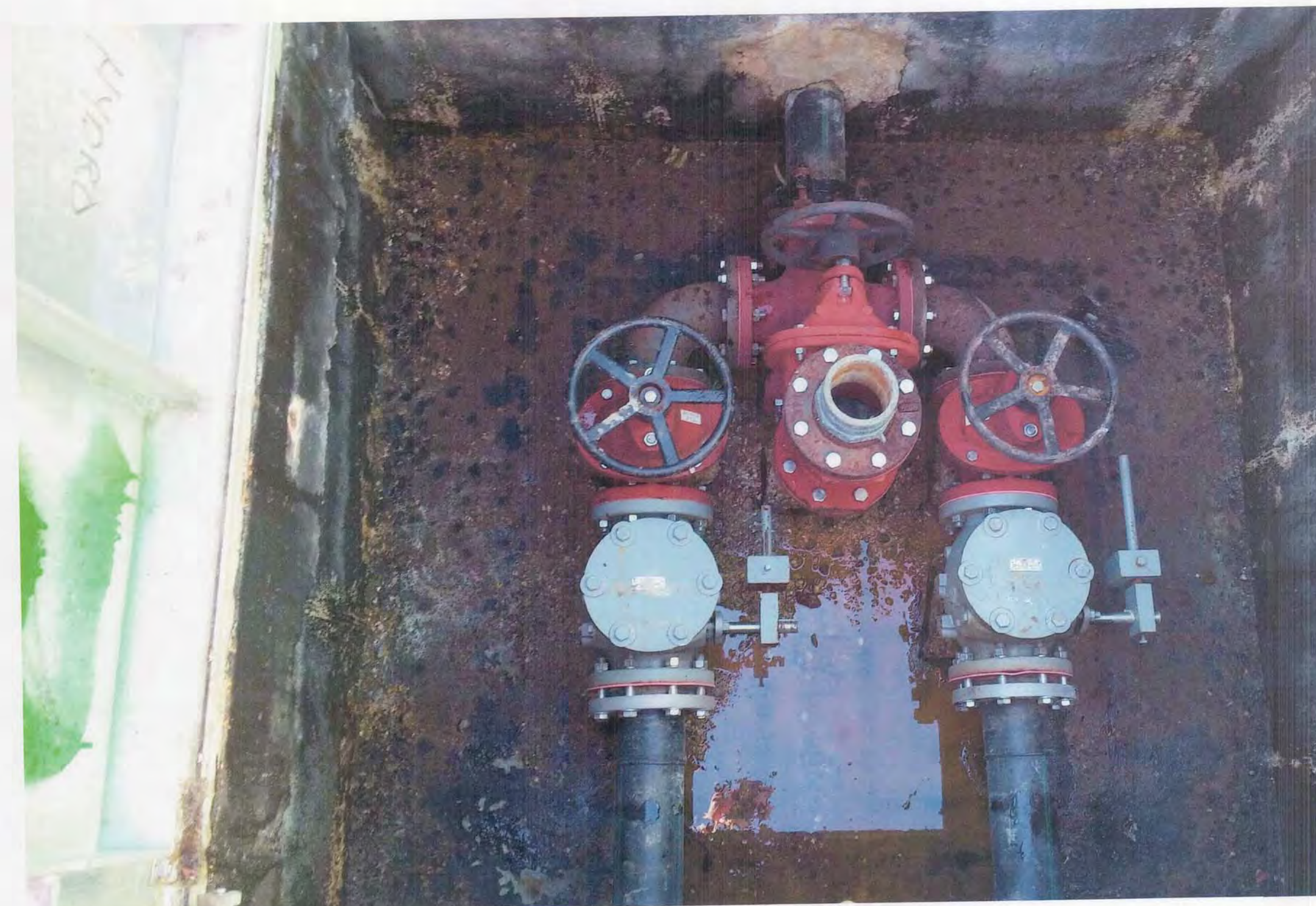
VALVE VAULT (RECOAT)
