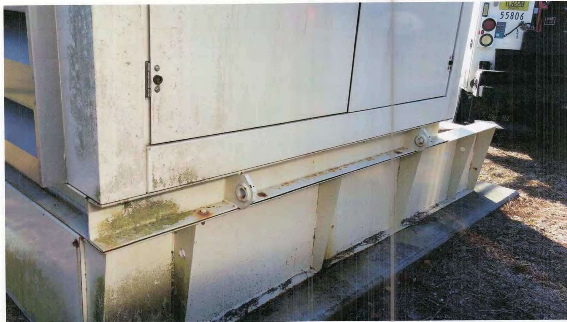
GENERATOR AND FUEL TANK REHABILITATION
