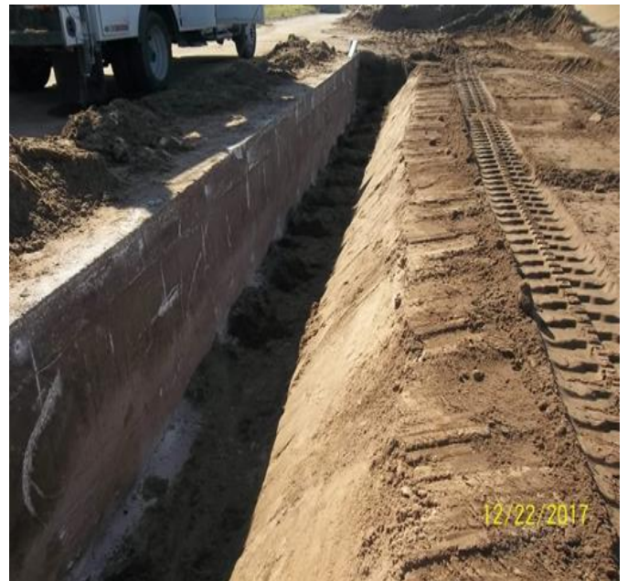
Spreader Ditch – Anchor Trench
