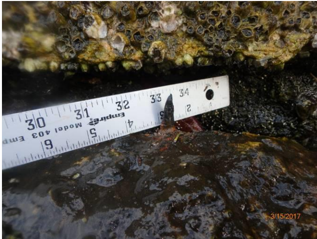
Photo #9 Panel 17, damaged area crack with exposed rebar
