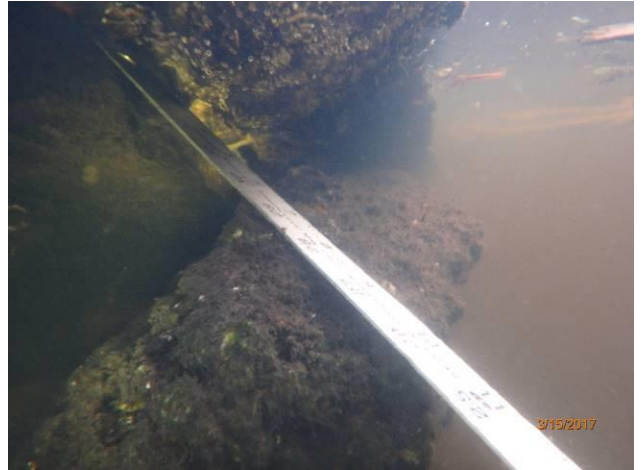
Photo #6 West end of damaged area panel 9 bukled
