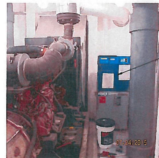
EXISTING DAY TANK (TO BE REMOVED)
