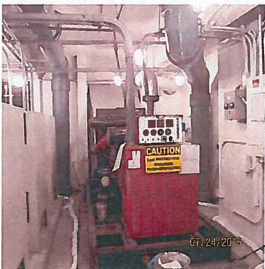
EXISTING GENERATOR (TO BE REMOVED)
