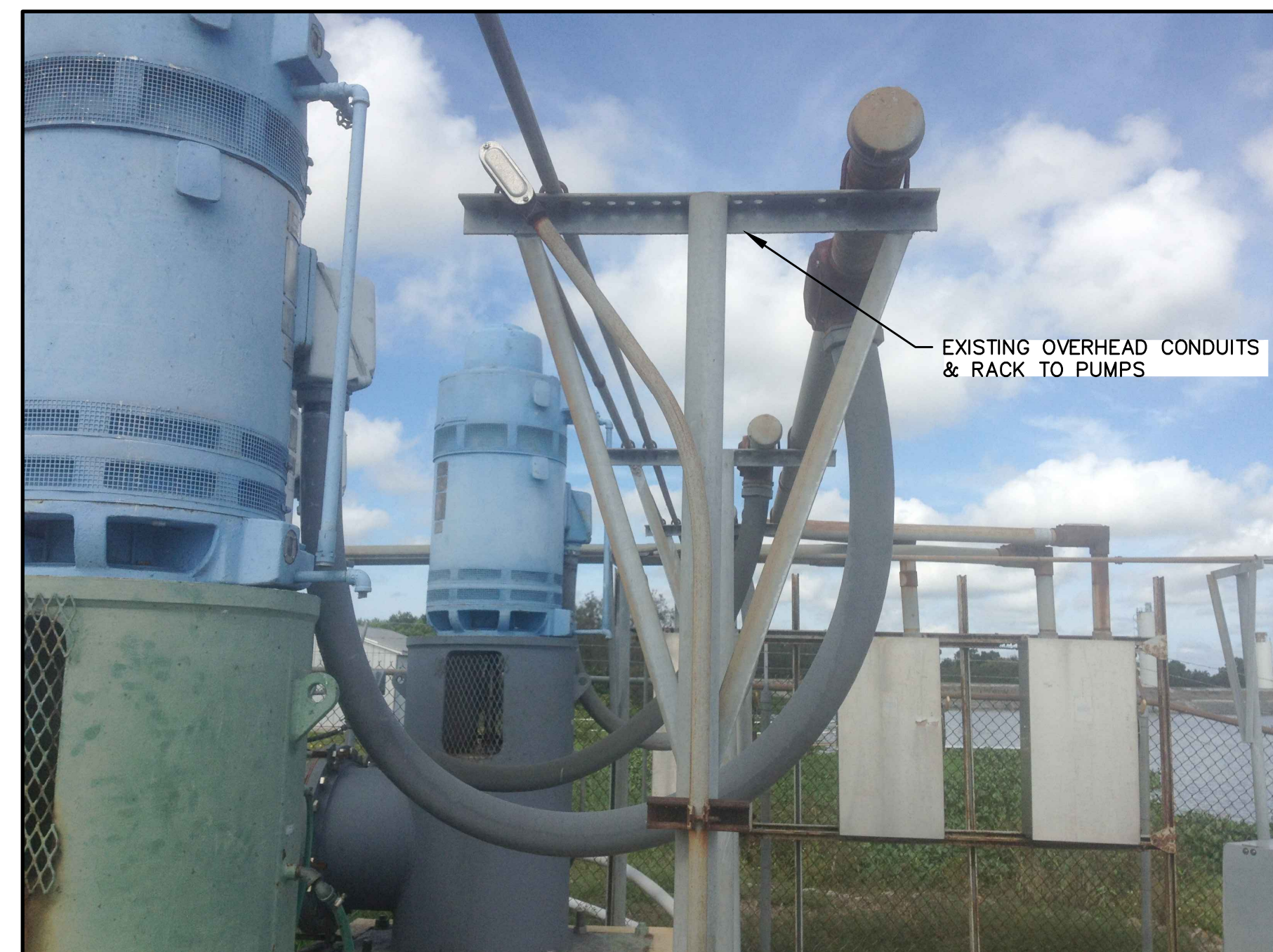
PHOTO 1 NTS EXISTING PUMPS AND DISCONNECTS
