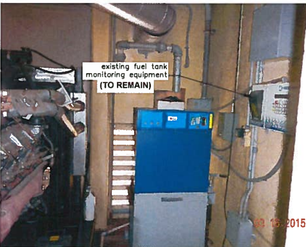
EXISTING DAY TANK (TANK, FUEL LINES, VENT, ETC.) TO BE REMOVED
