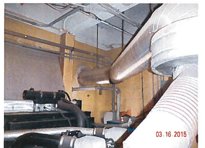
EXISTING GENERATOR EXHAUST DUCT (TO BE REMOVED)
