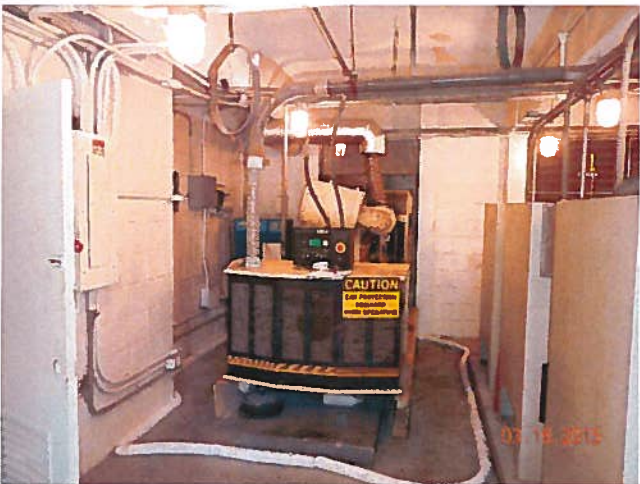
EXISTING GENERATOR (TO BE REMOVED)
