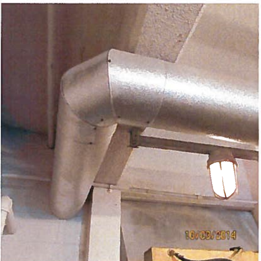
EXISTING GENERATOR EXHAUST DUCT (TO BE REMOVED)
