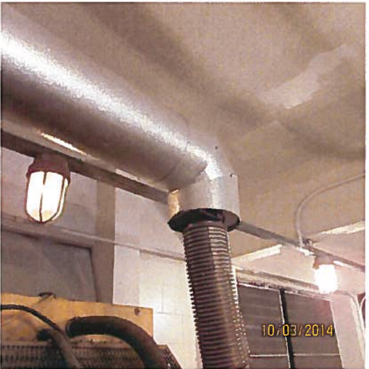
EXISTING GENERATOR EXHAUST DUCT (TO BE REMOVED)
