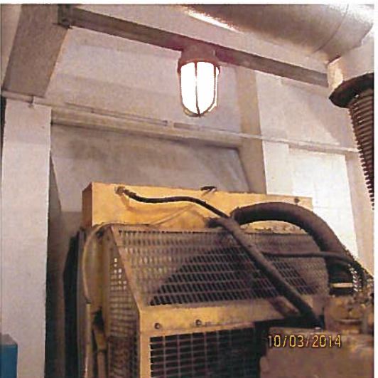
EXISTING GENERATOR RADIATOR AND DUCT (TO BE REMOVED)
