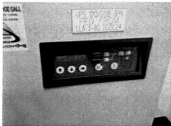
Figure 1: Existing Chloride UPS System
