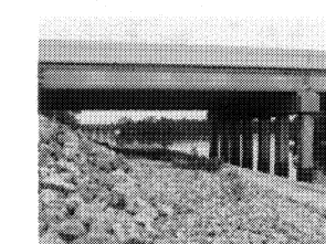
BENEATH BRIDGE SOUTH VIEW
