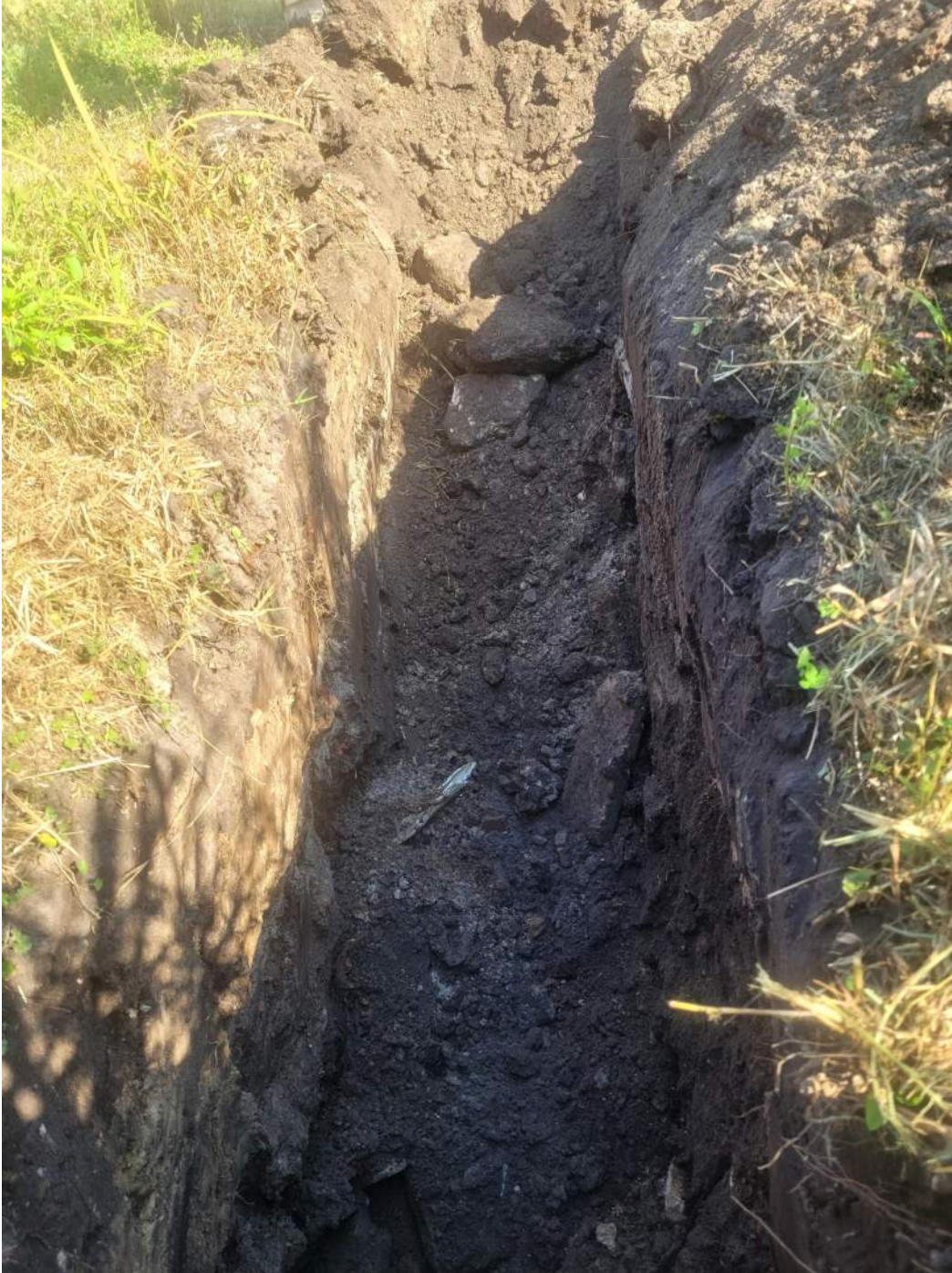
Photograph 5. Test Pit TP-4
