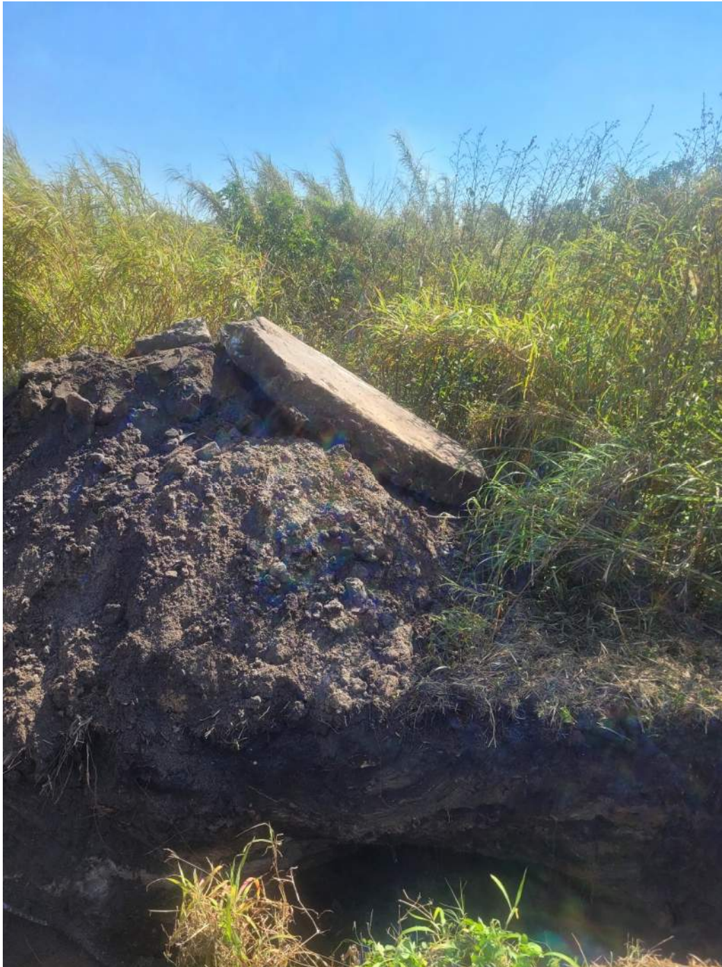
Photograph 6. Test Pit TP-4.
