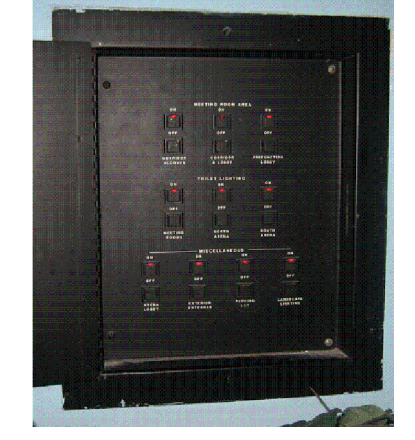
PICTURE OF EXISTING PANEL. REPLACE CONTROL SURFACE NEW SURFACE TO HAVE (4) PAIRS OF (2) BUTTONS, (4) "ON" BUTTONS TO HAVE PILOT LIGHTS. BUTTONS WILL CONTROL "ARENA LOBBY", "EXTERIOR ENTRANCE", "PARKING LOT", AND "LANDSCAPE LIGHTING" AS SHOWN TO THE LEFT.
