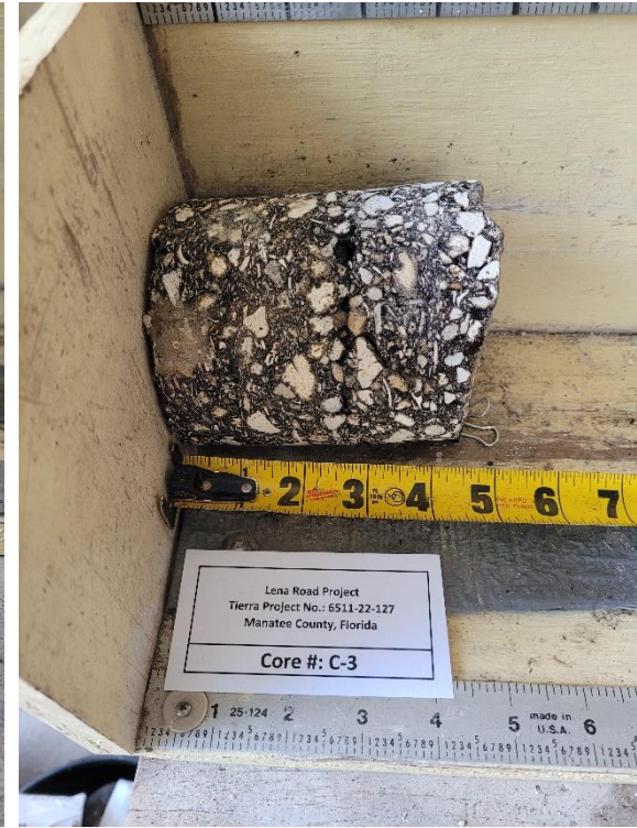
Photograph 9. Pavement Core No. C-3 Side View
