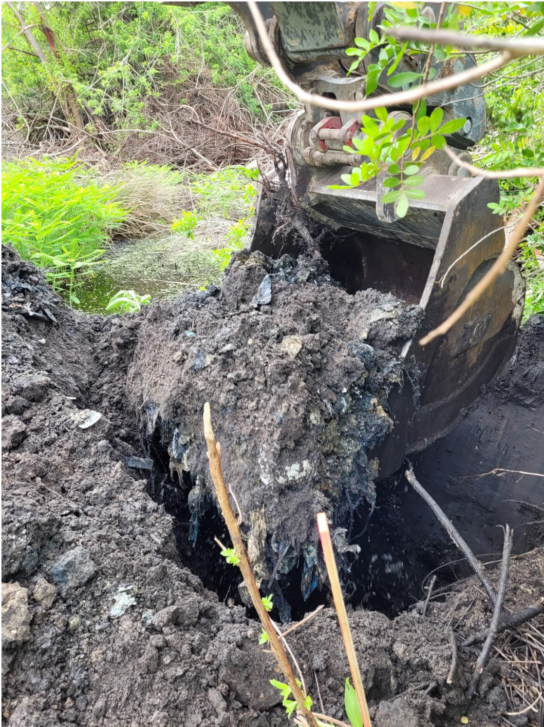
Test Pit TP-21
