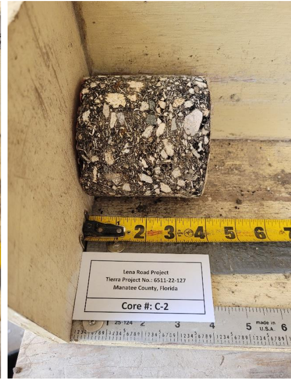
Photograph 6. Pavement Core No. C-2 Side View
