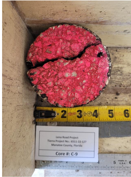
Photograph 26. Pavement Core No. C-9 Top View
