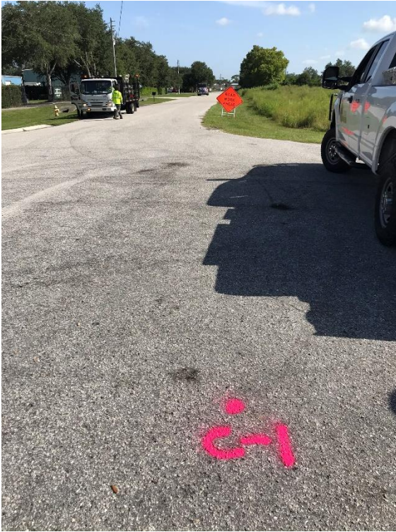
Photograph 1. Pavement Core No. C-1 Field
