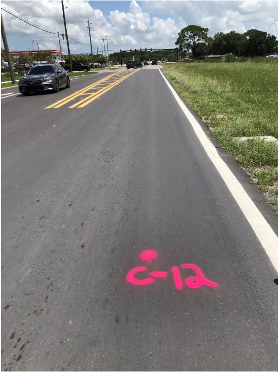
Photograph 34. Pavement Core No. C-12 Field
