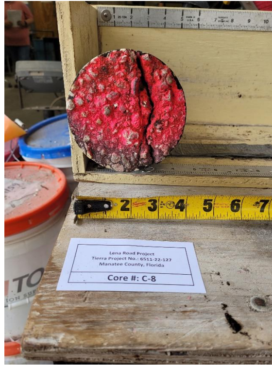
Photograph 23. Pavement Core No. C-8 Top View
