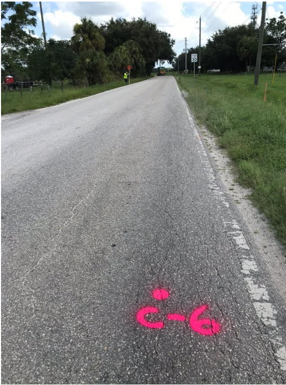
Photograph 16. Pavement Core No. C-6 Field
