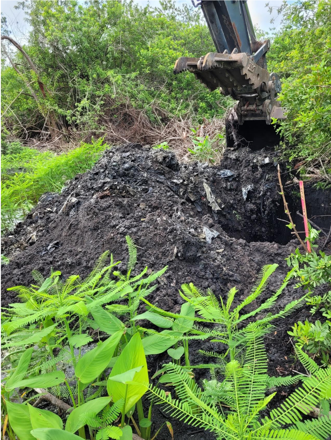
Test Pit TP-21
