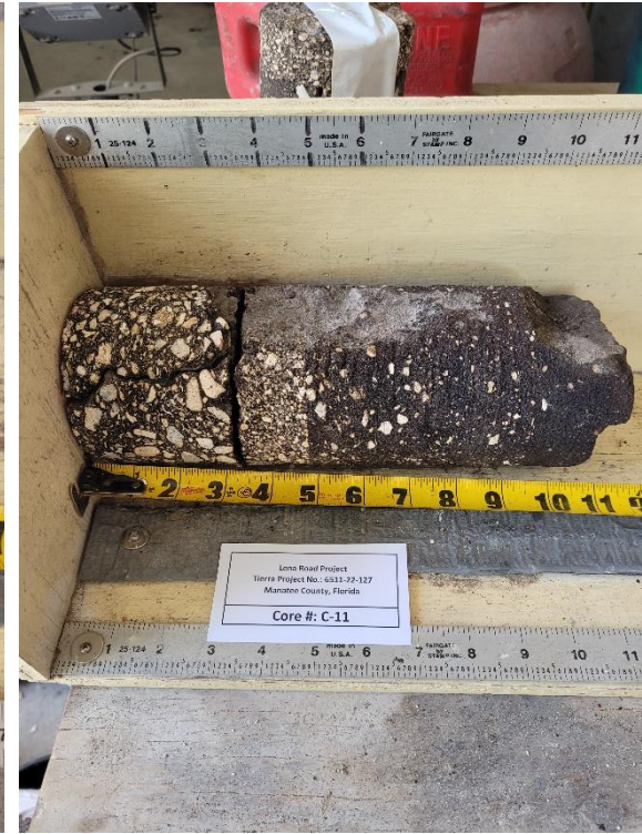
Photograph 33. Pavement Core No. C-11 Side View
