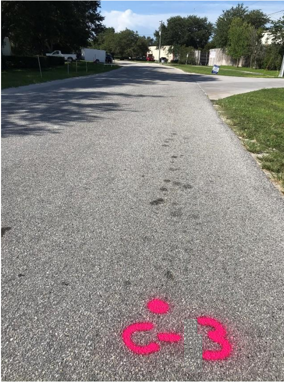
Photograph 7. Pavement Core No. C-3 Field
