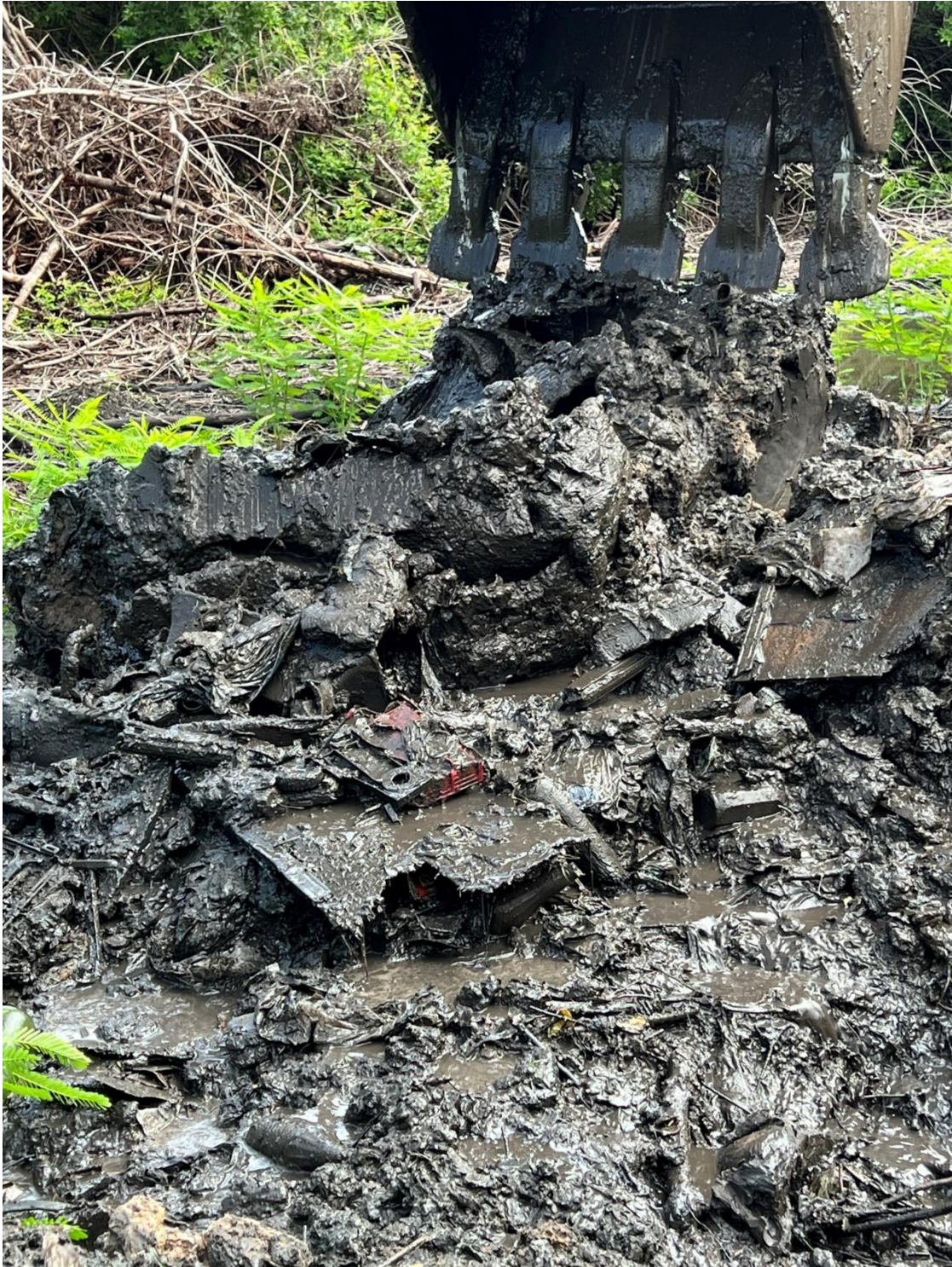
Test Pit TP-15
