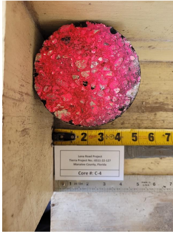
Photograph 11. Pavement Core No. C-4 Top View
