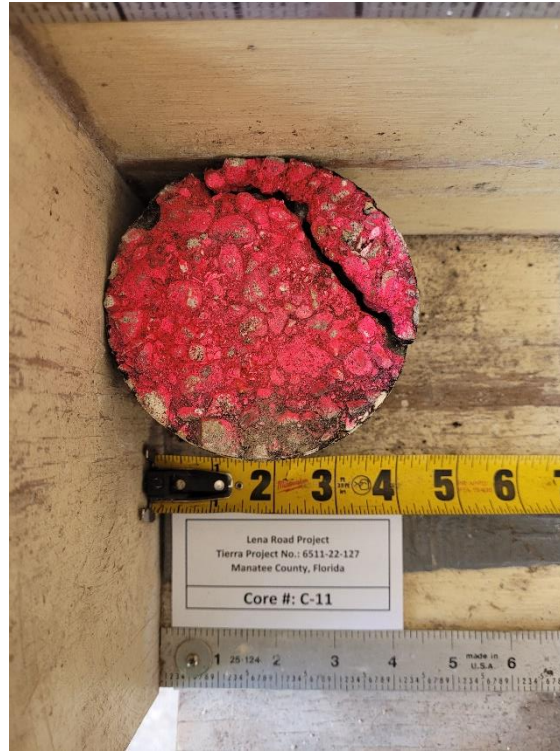
Photograph 32. Pavement Core No. C-11 Top View
