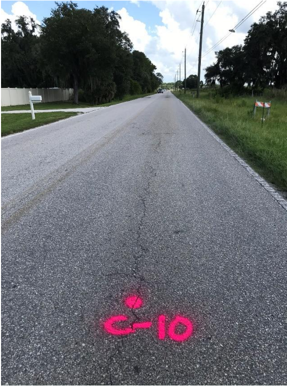
Photograph 28. Pavement Core No. C-10 Field
