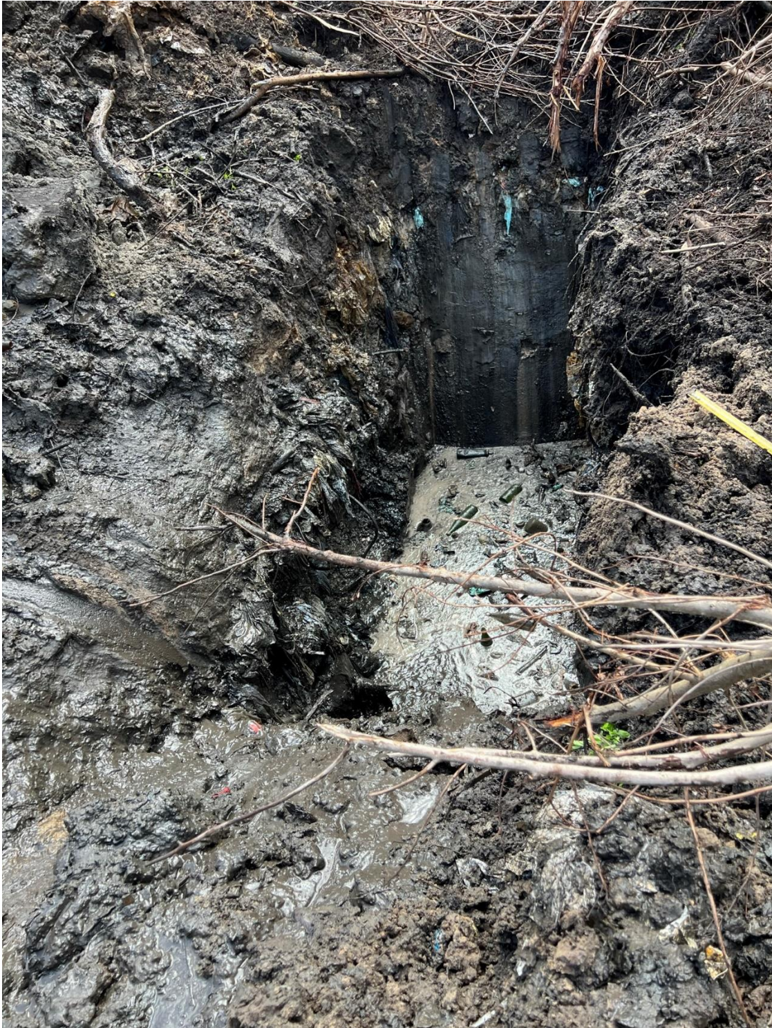
Test Pit TP-15
