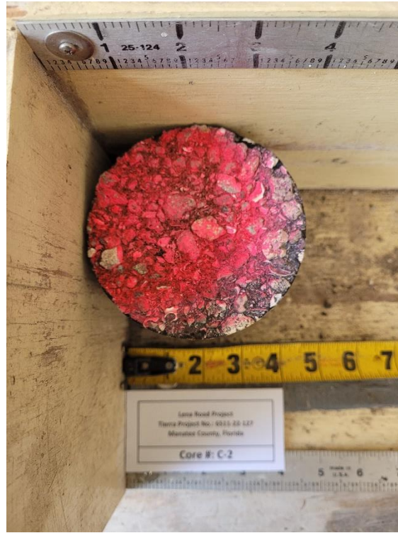
Photograph 5. Pavement Core No. C-2 Top View
