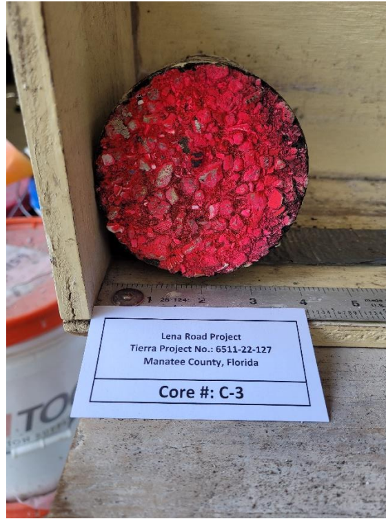
Photograph 8. Pavement Core No. C-3 Top View
