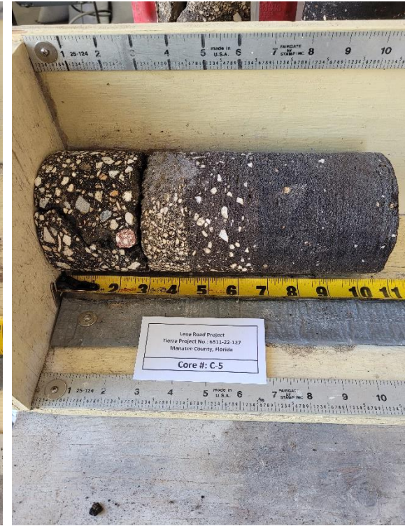
Photograph 15. Pavement Core No. C-5 Side View
