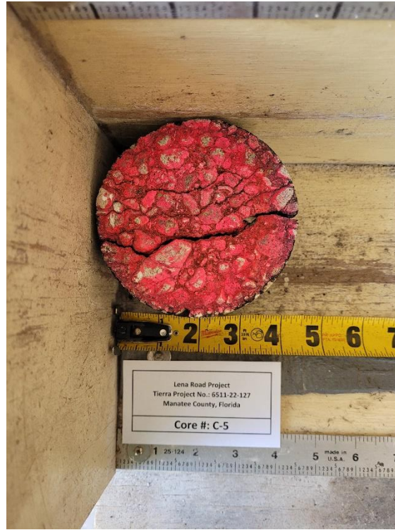
Photograph 14. Pavement Core No. C-5 Top View
