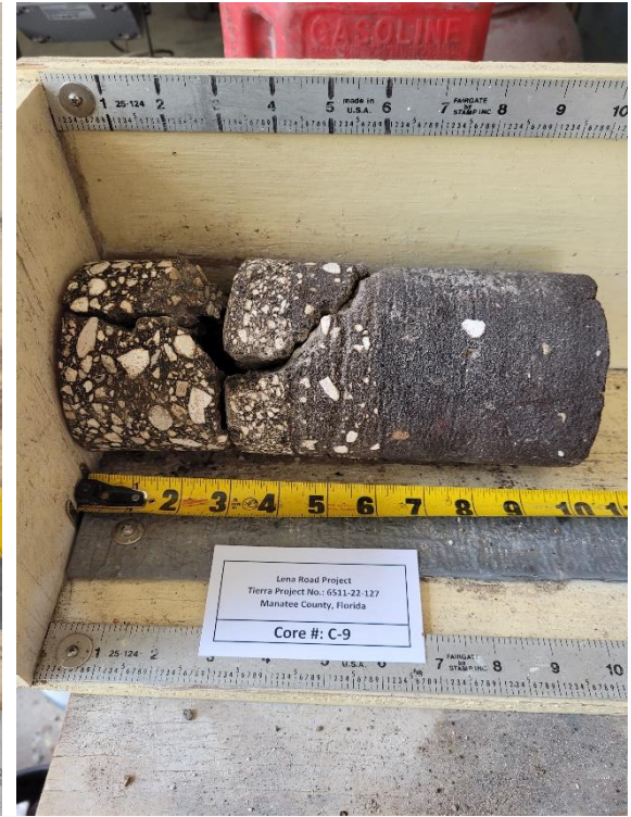
Photograph 27. Pavement Core No. C-9 Side View
