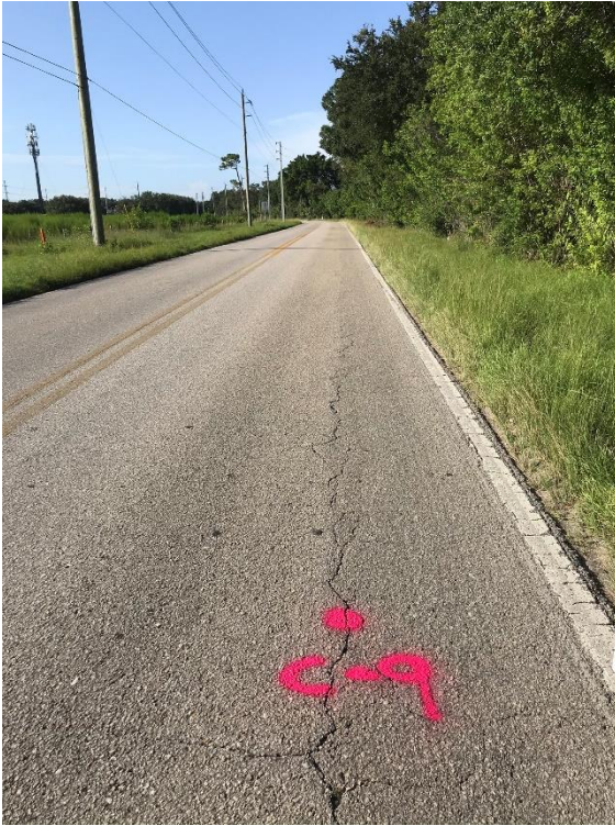
Photograph 25. Pavement Core No. C-9 Field
