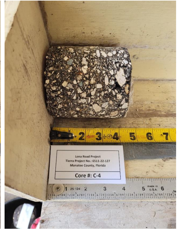
Photograph 12. Pavement Core No. C-4 Side View
