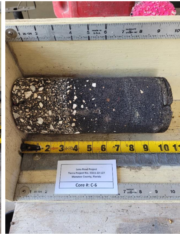
Photograph 18. Pavement Core No. C-6 Side View
