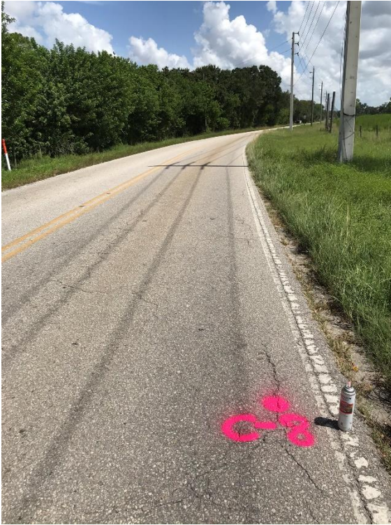
Photograph 22. Pavement Core No. C-8 Field
