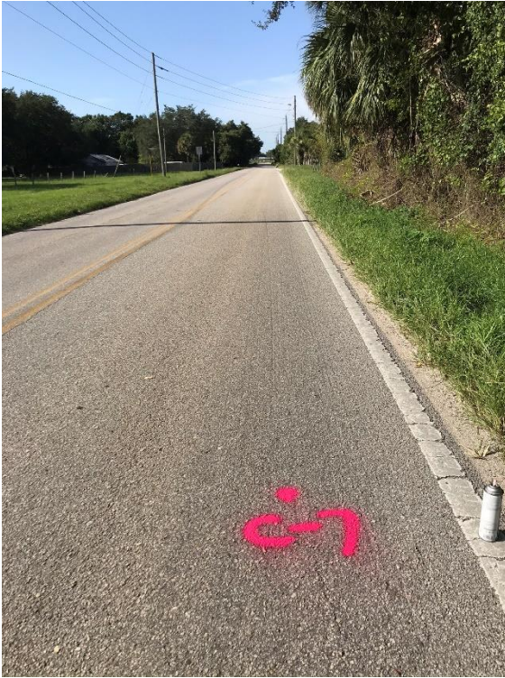
Photograph 19. Pavement Core No. C-7 Field
