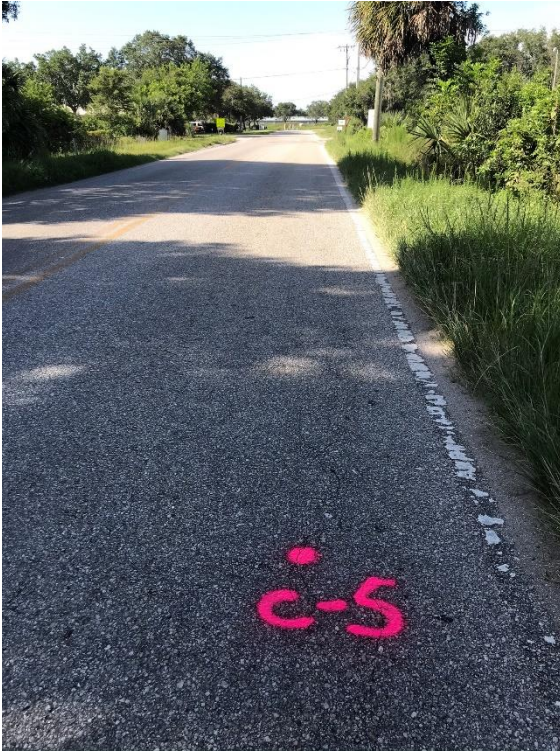
Photograph 13. Pavement Core No. C-5 Field
