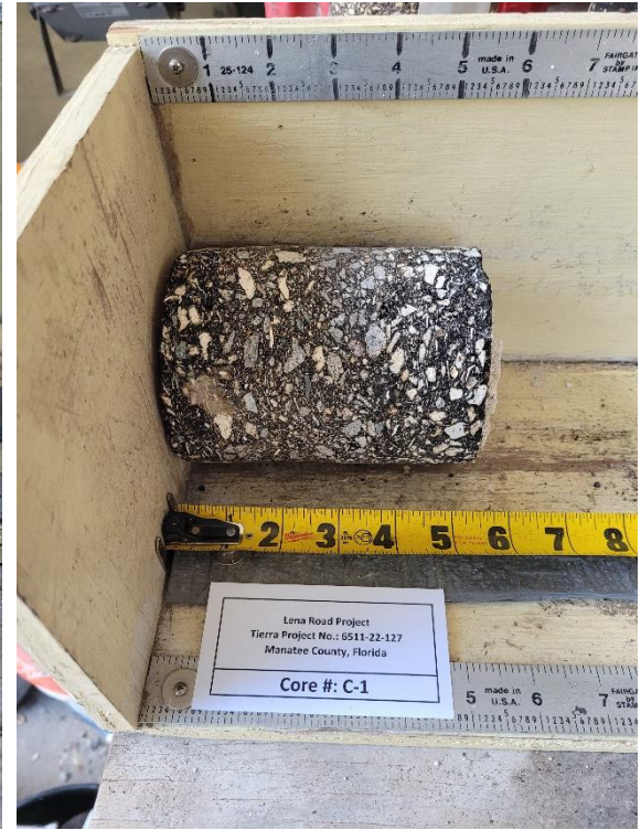
Photograph 3. Pavement Core No. C-1 Side View
