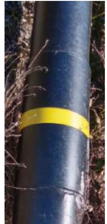
FIG. 3 POLE WEEDEATER GUARD WITH TAPE LINE
