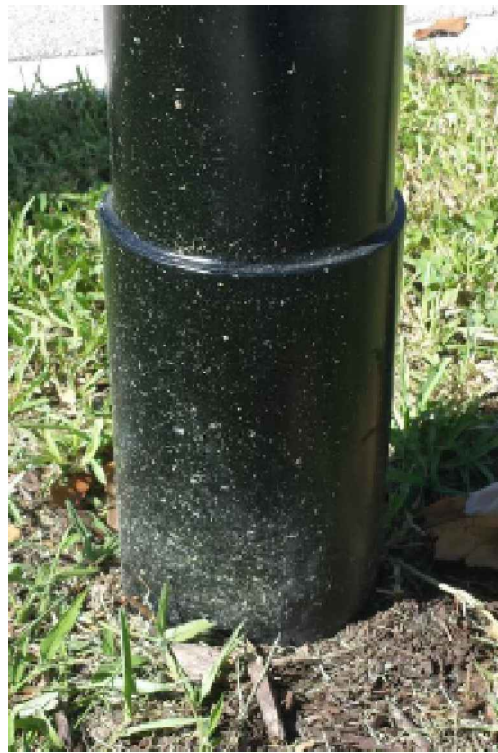
FIG.2 PROPER EMBEDMENT TO TAPE LINE
