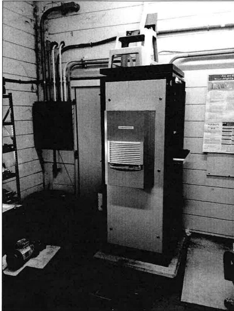
REPLACE EXISTING ANALOG TERMINATION CABINET FOR DCU-3
