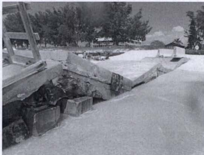
Figure 2. Existing deteriorated middle groin
