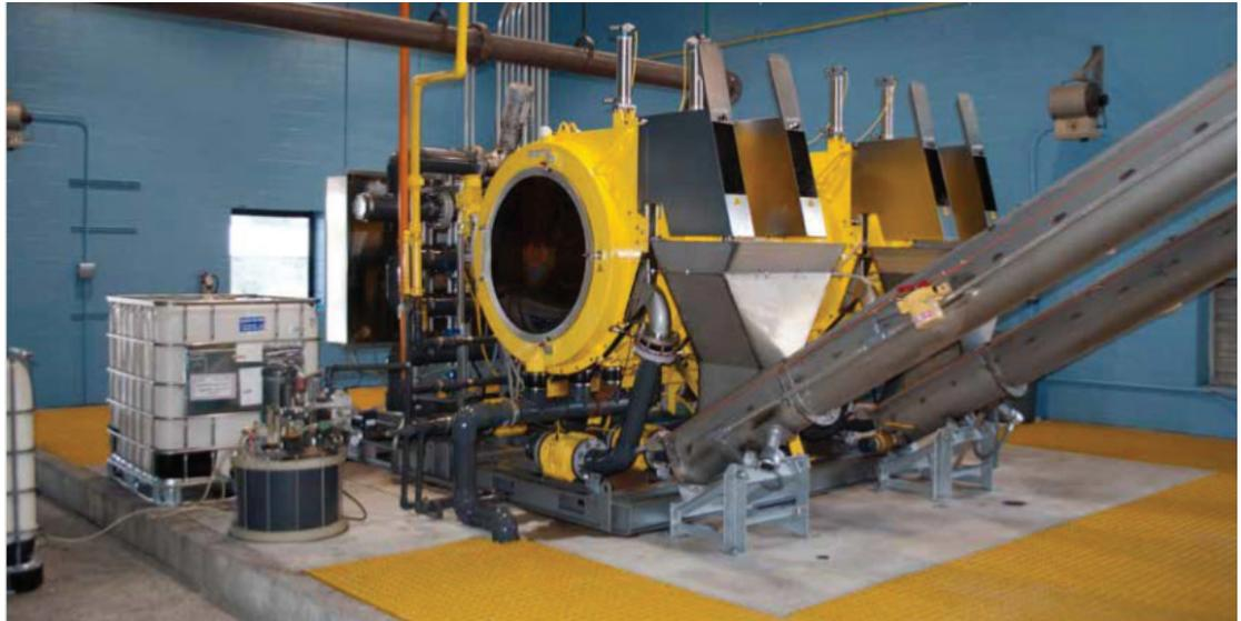
Figure 19 Rotary Fan Press Installation (Madisonville, KY, West Side WWTP)
