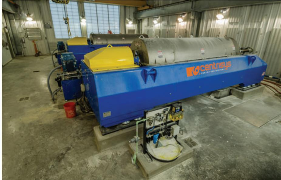
Figure 14 Typical Centrifuge Installation
