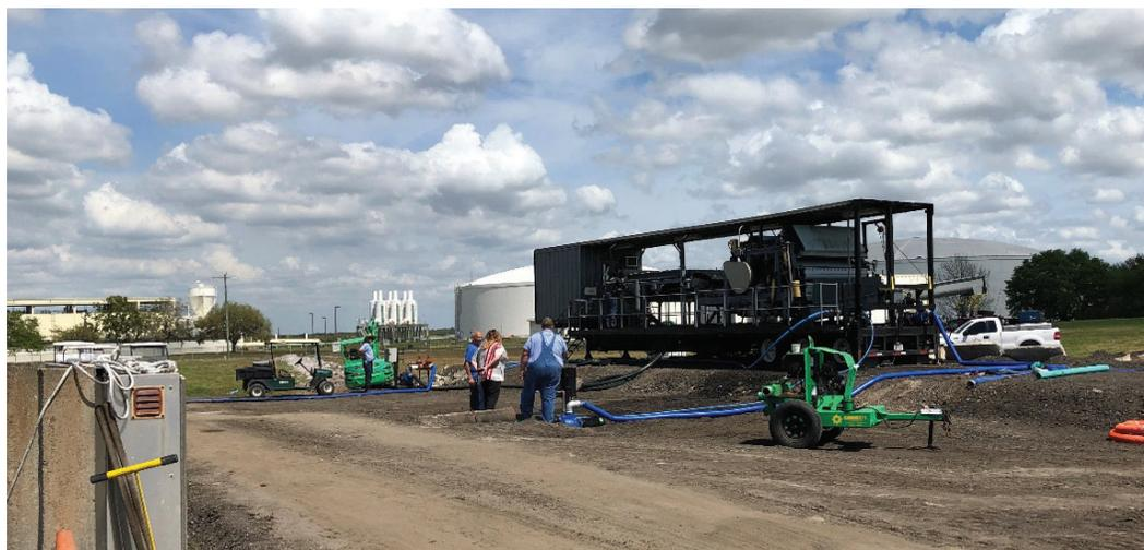
Figure 1 Temporary Belt Filter Press
