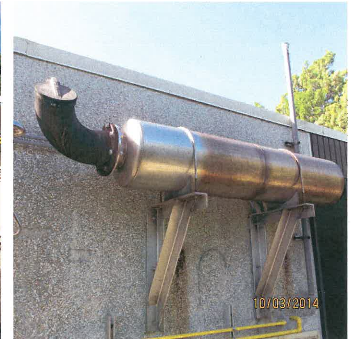
EXISTING GENERATOR MUFFLER - TO BE REMOVED (FACING SOUTH WEST)
