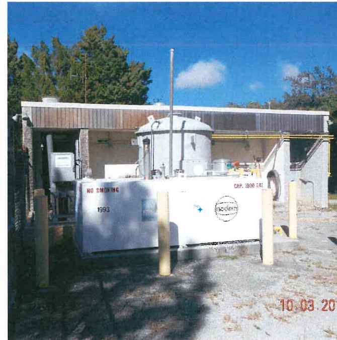
EXISTING DIESEL TANK - TO BE REMOVED (FACING WEST)
