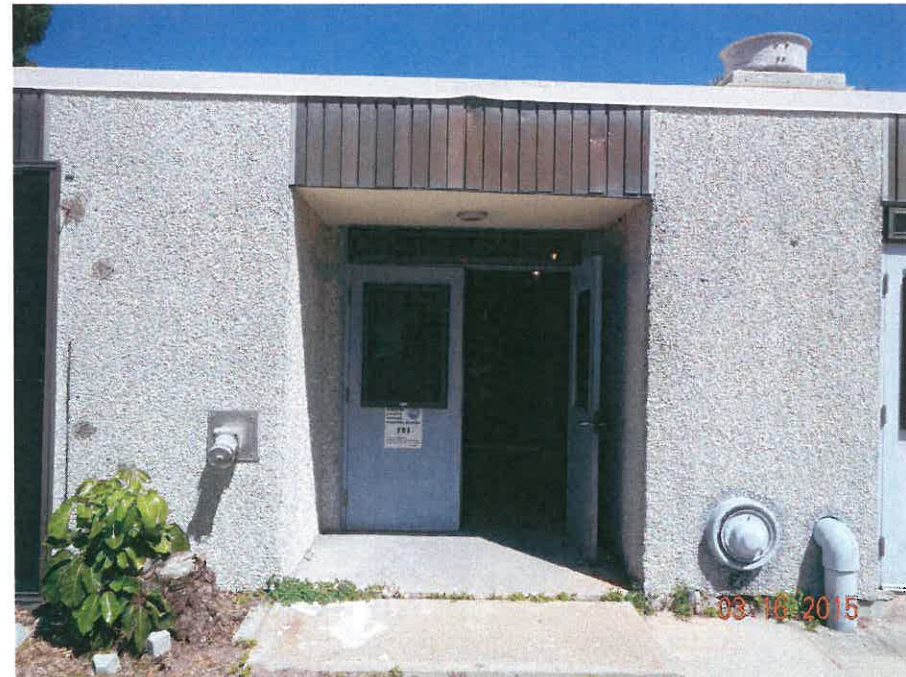
BUILDING MAIN ENTRY (FACING NORTH)
