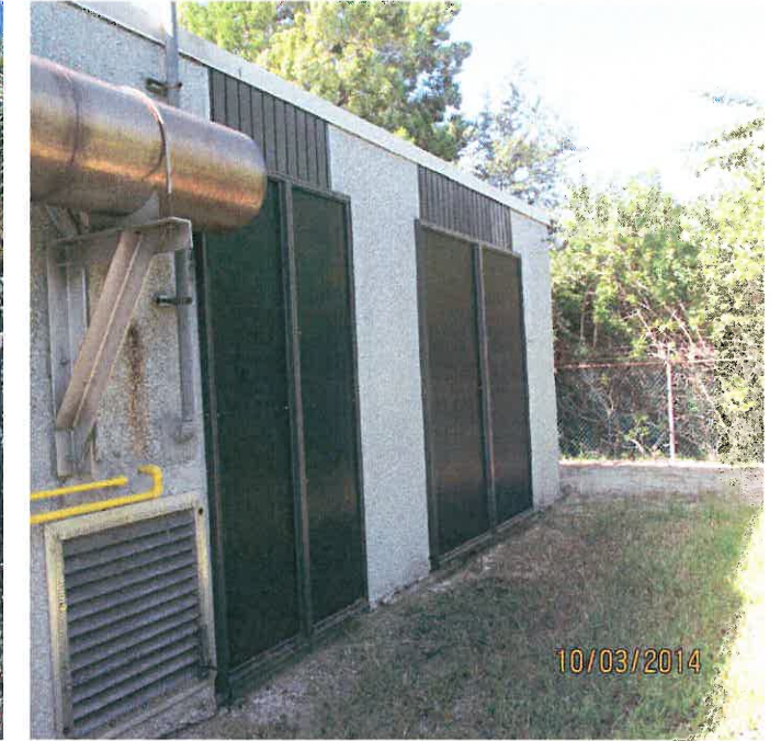
SITE PHOTO (FACING SOUTHWEST)
