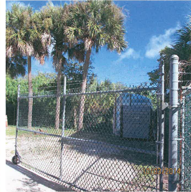
SITE PHOTO (FACING NORTH)
