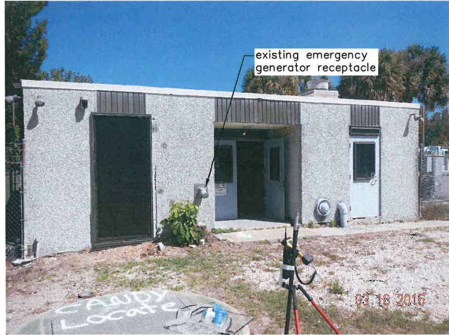
EXISTING BUILDING (FACING NORTH)
