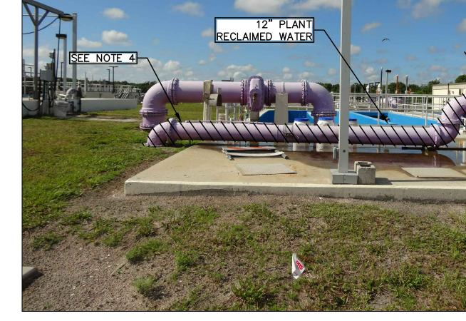
4. CONTRACTOR SHALL REMOVE 12" PLANT WATER FEED TO 3 FEET BELOW GRADE AND CAP LINE.
