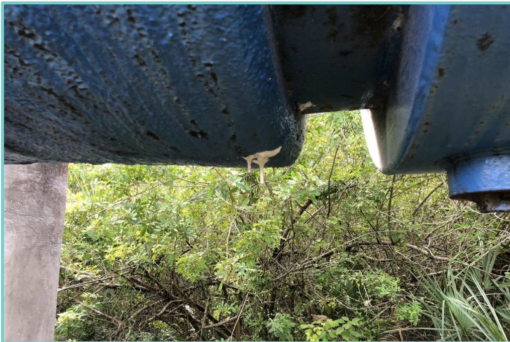
Photo 2-4 – Calcified stalagmite growth at joints
