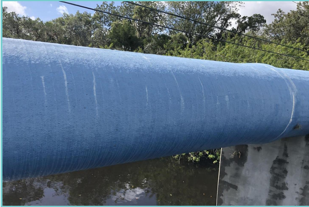
Photo 2-3 – Typical mortar cracks in 42" PWM surface
