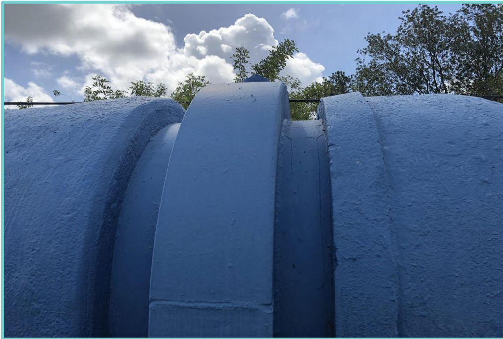
Photo 2-2 – Past joint repair at 42" PWM
