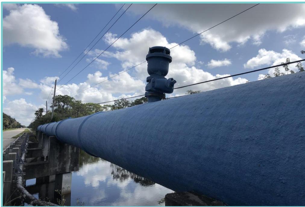
Photo 2-1 – 42" PWM Spanning Mill Creek South of Bridge No. 134023
