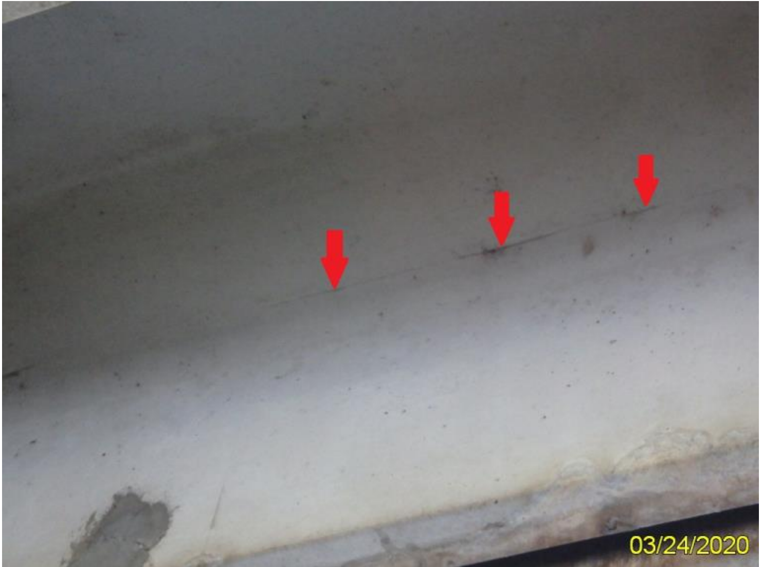
Photo 8 - Element 109 Pre Opn Conc Girder/Beam
