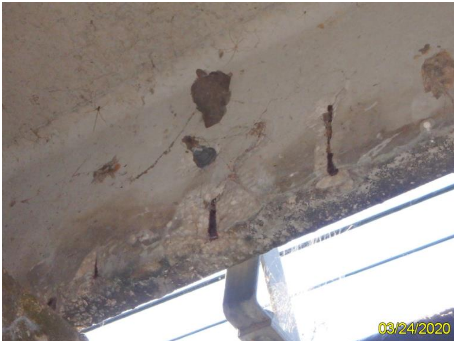
Photo 2 - Element 109 Pre opn Conc Girder/Beam
