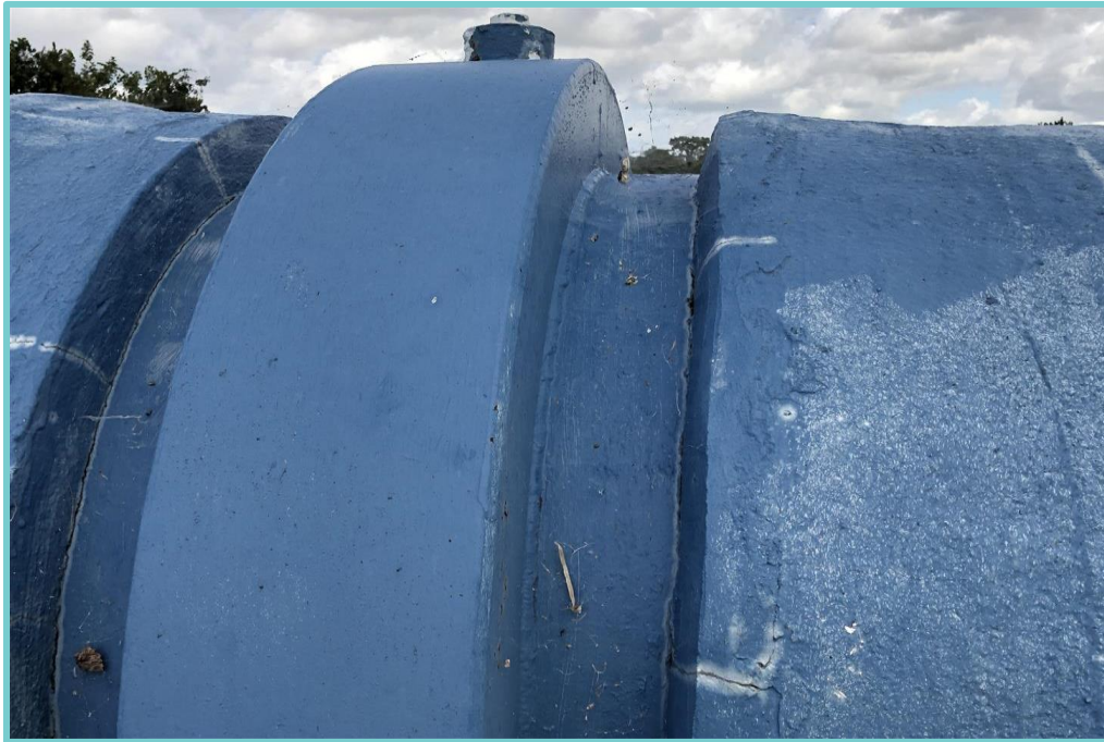
Photo 2-2 – Past joint repair at 42" PWM
