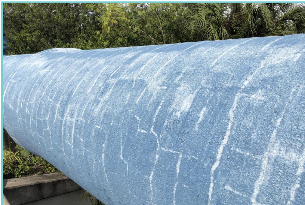
Photo 2-3 – Typical mortar cracks in 42" PWM surface
