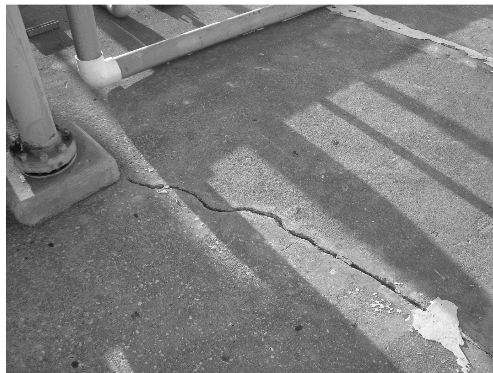
C REPAIR CRACKS IN CONCRETE
