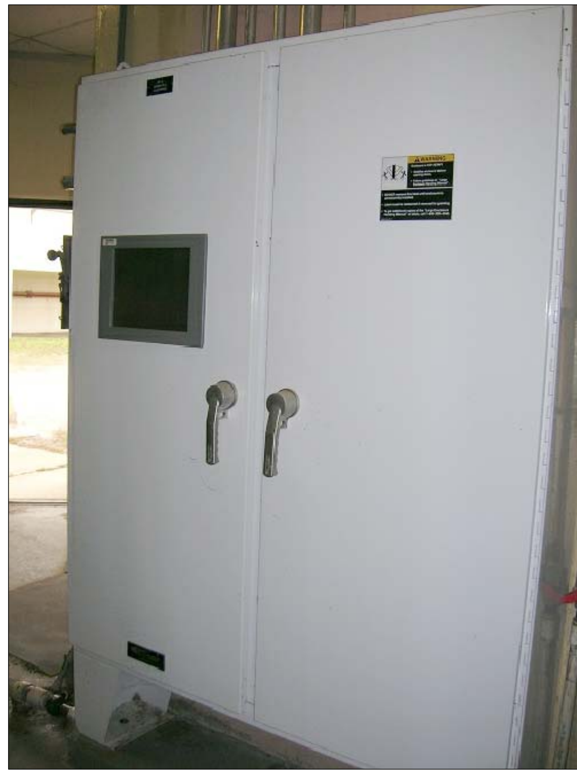
EXISTING HEADWORKS PLC PANEL NOT TO SCALE
