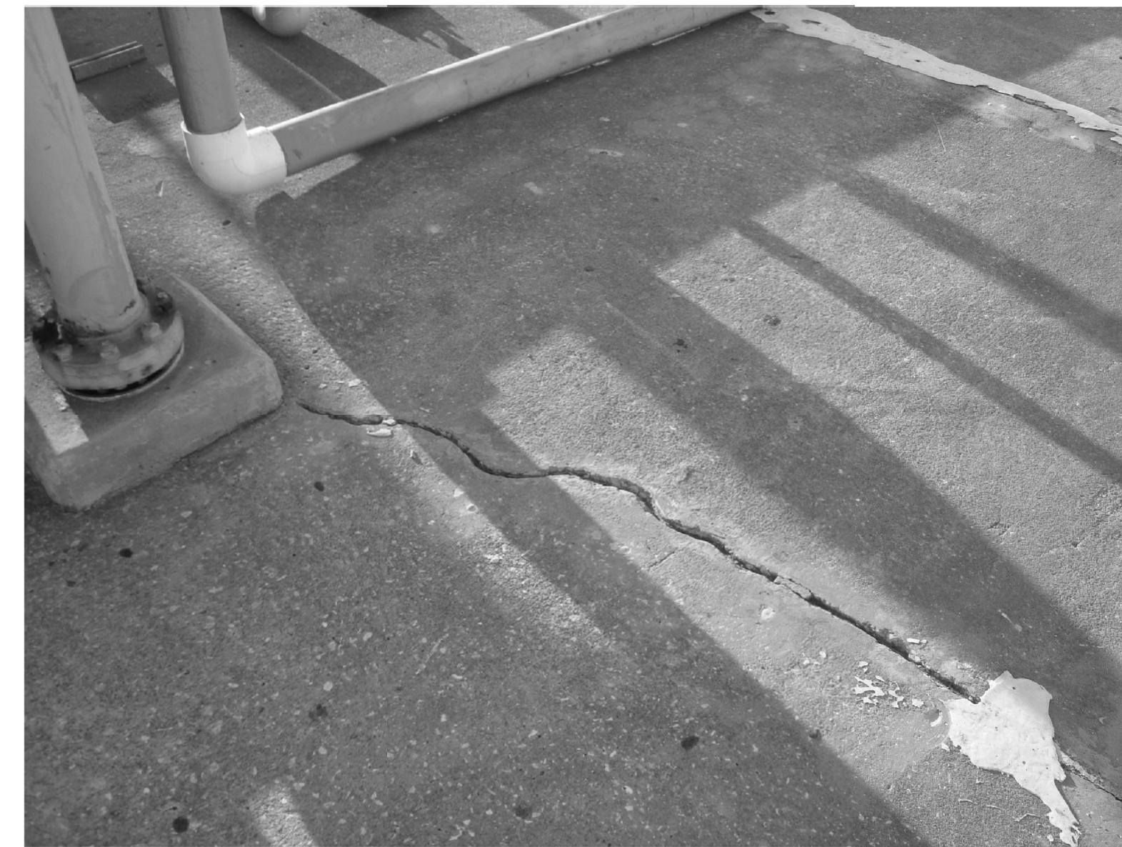
C REPAIR CRACKS IN CONCRETE
