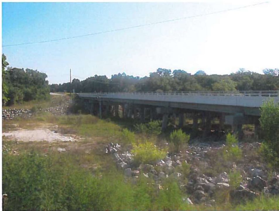
Bridge #134114 (previously #134022) looking northeast.
