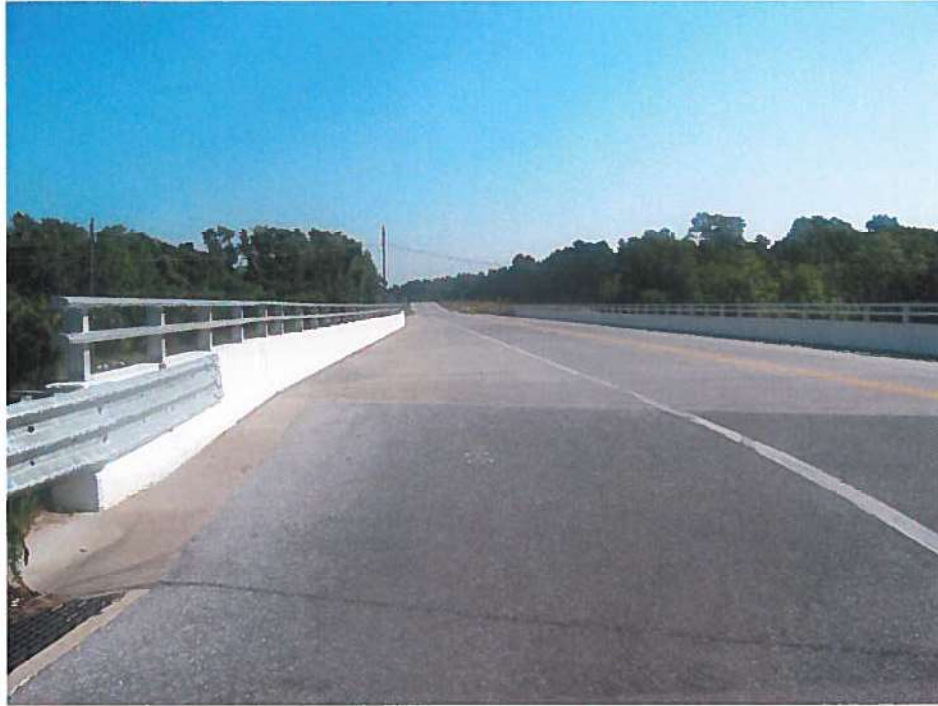
Bridge #134114 (previously #134022) looking north.
