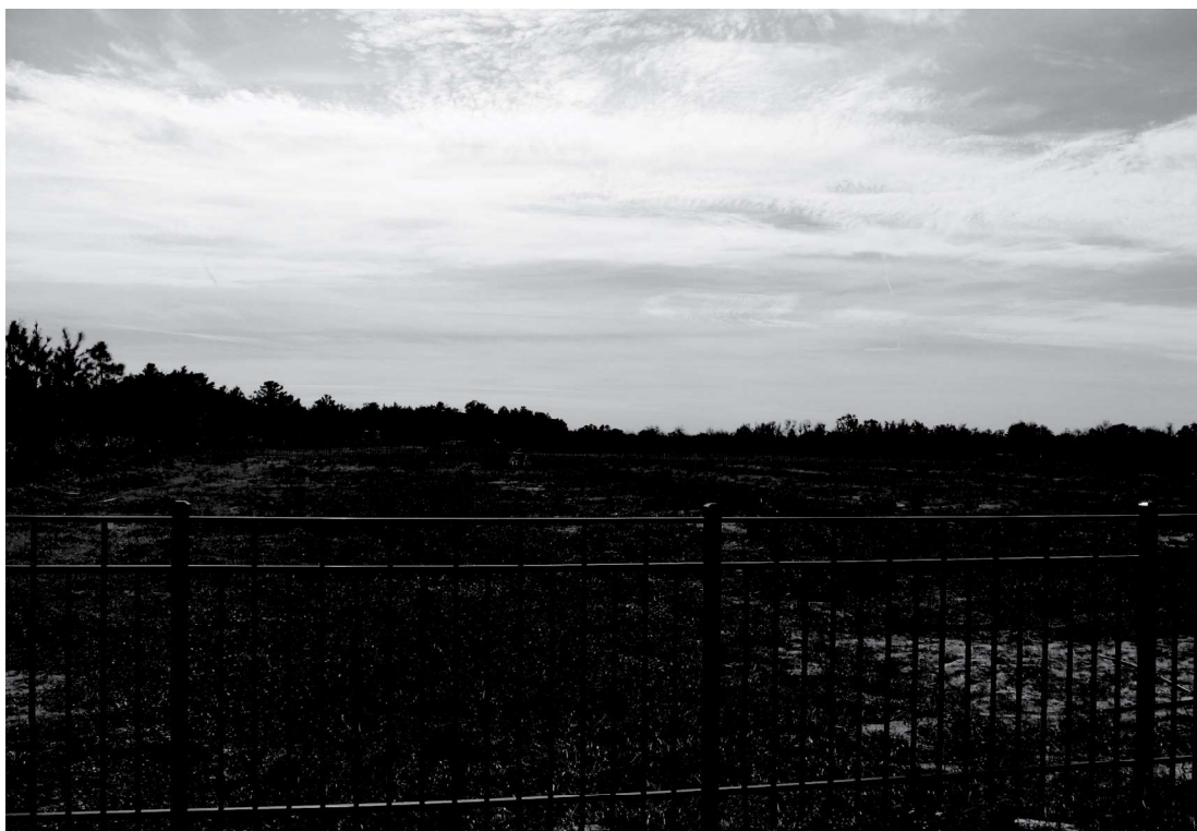
Newly installed fence surrounding cemetery and grave marker west of Rye Road
