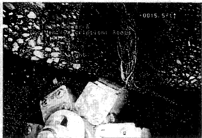
R - Roots @ 15.5 ft. light in joint
