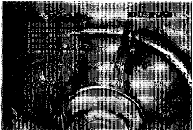
R - Roots @ 148.2 ft. medium from joint
