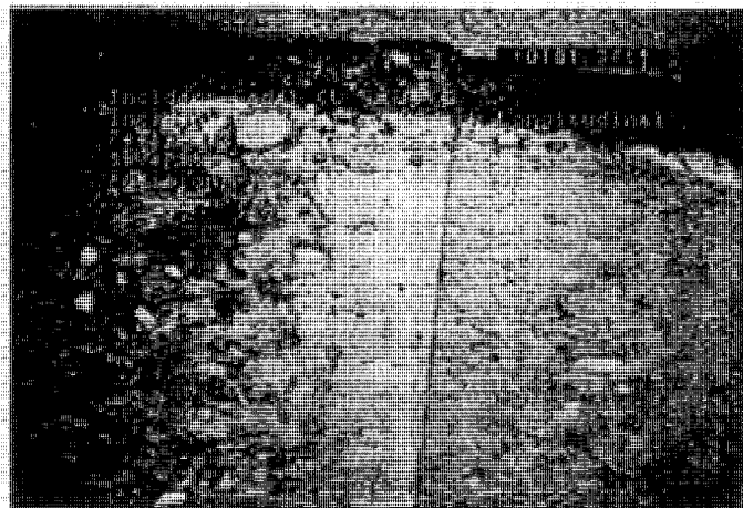
CL - Crack Longitudinal @ 181.3 ft.
