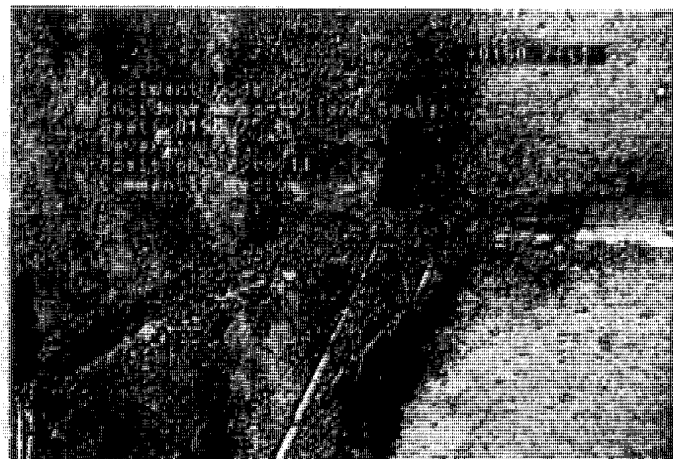
R - Roots @ 150.7 ft. medium in joint
