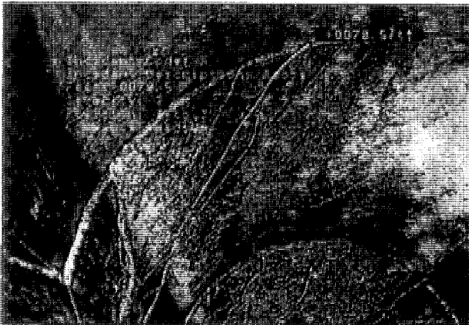
R - Roots @ 78.5 ft. medium from joint
