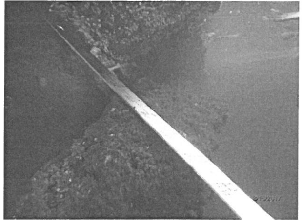
Photo #6 West end of damaged area panel 9 buckled
