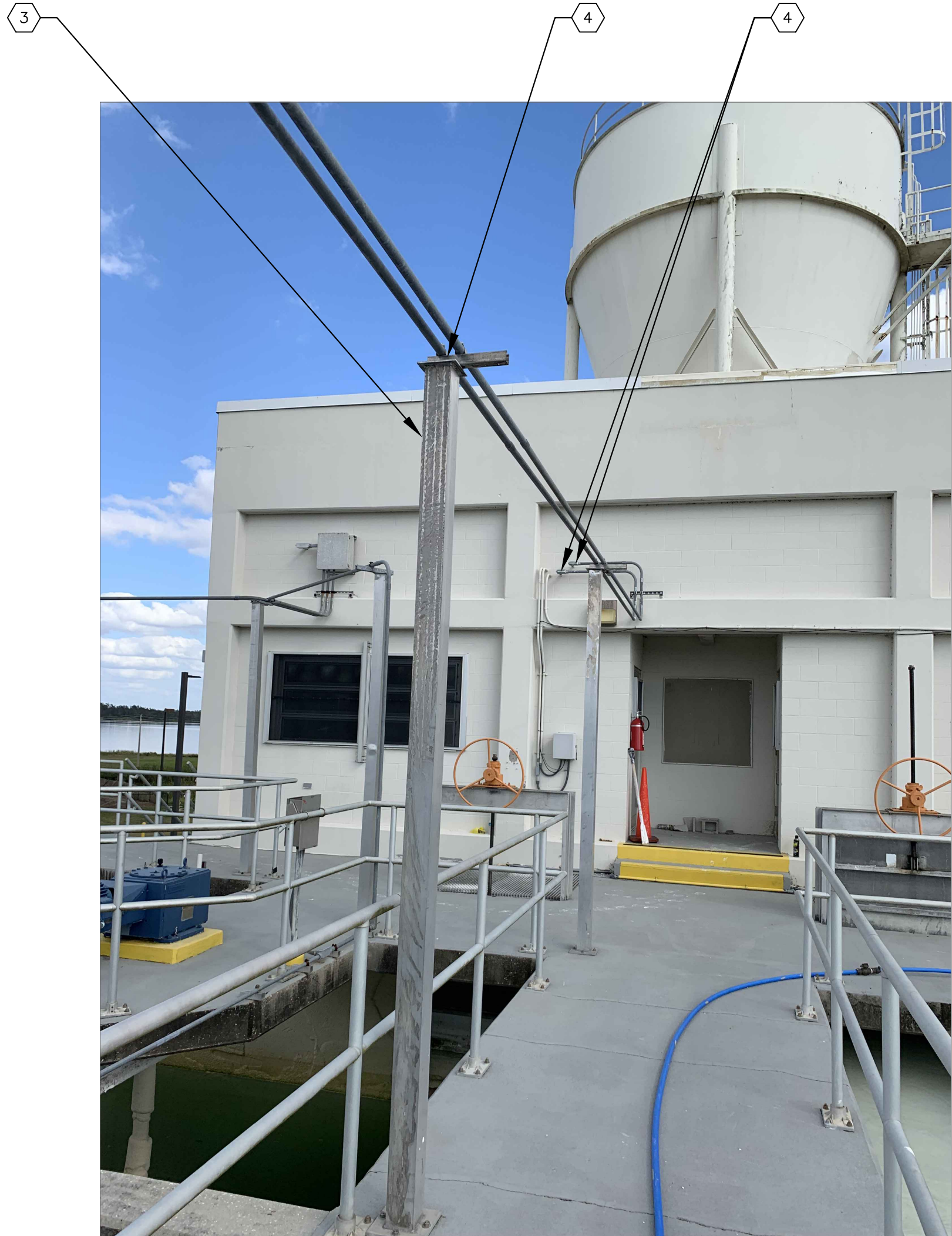
EXISTING CONDUIT SUPPORT ELEVATION
