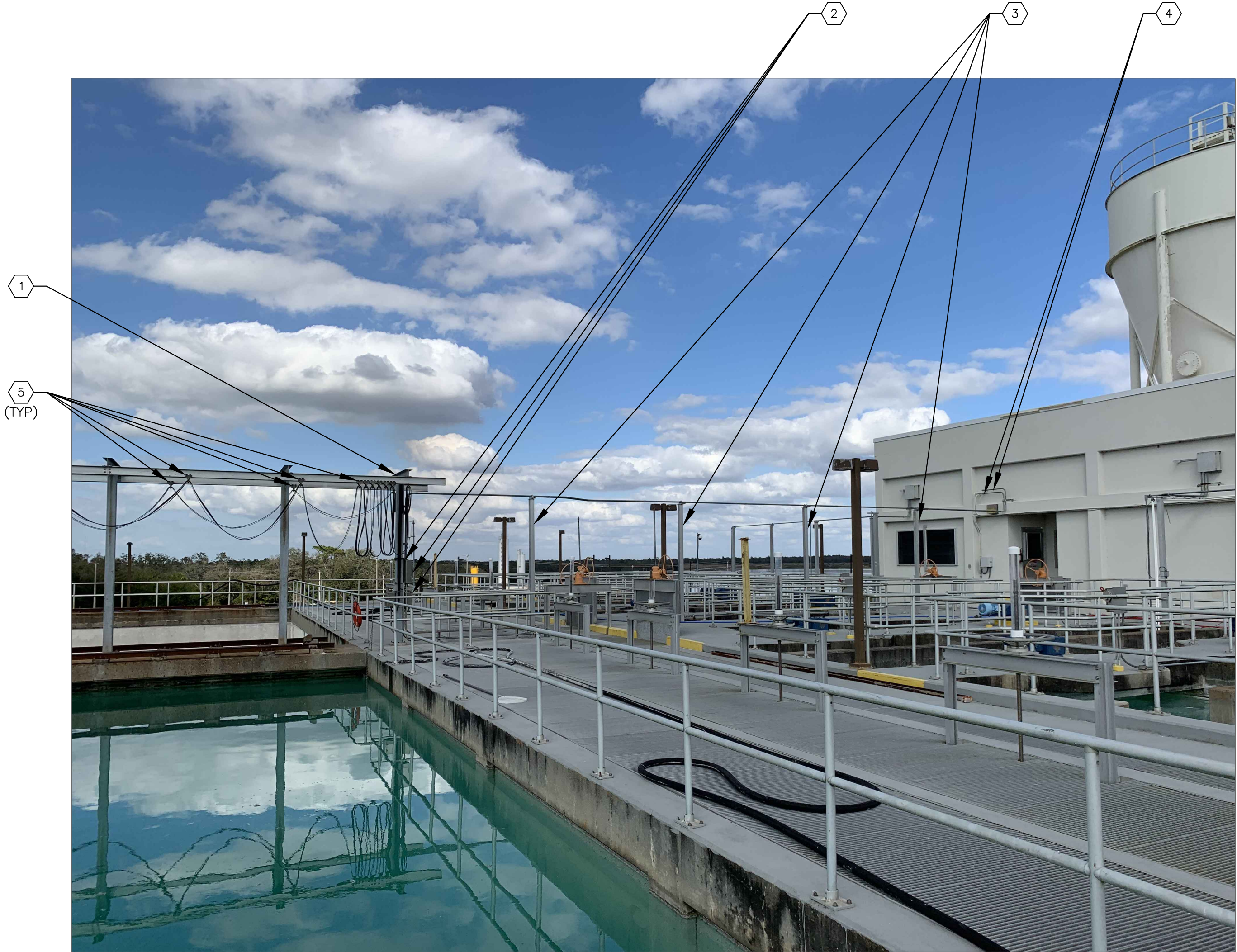
FESTOON AND EXISTING CONDUIT SUPPORT ELEVATION
