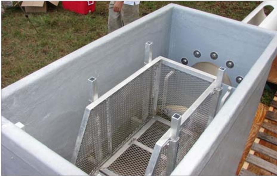
**Figure 1 - Sieve strainer screen of Type 2 baffle box**
