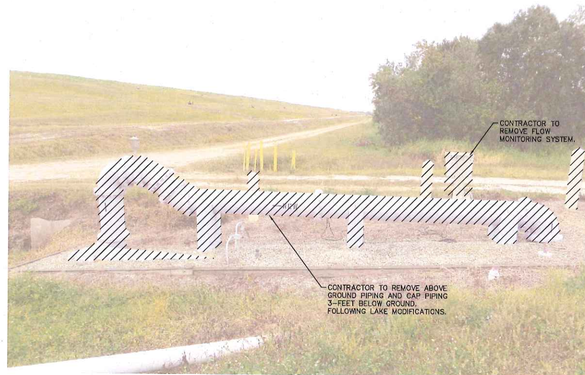
EX. EAST LAKE ABOVE GROUND PIPING
