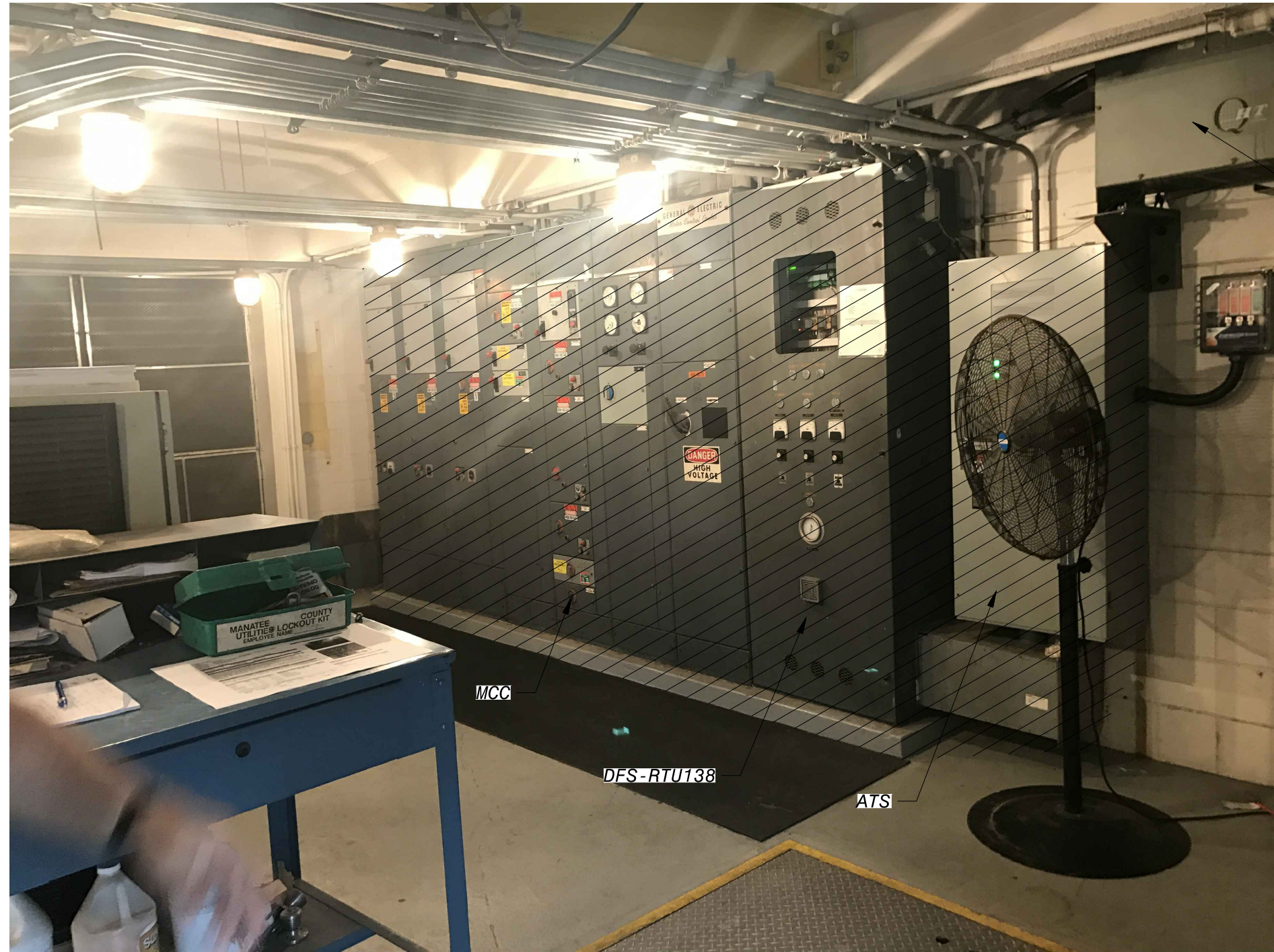
MCC, ATS, AND RTU DEMOLITION NO SCALE
