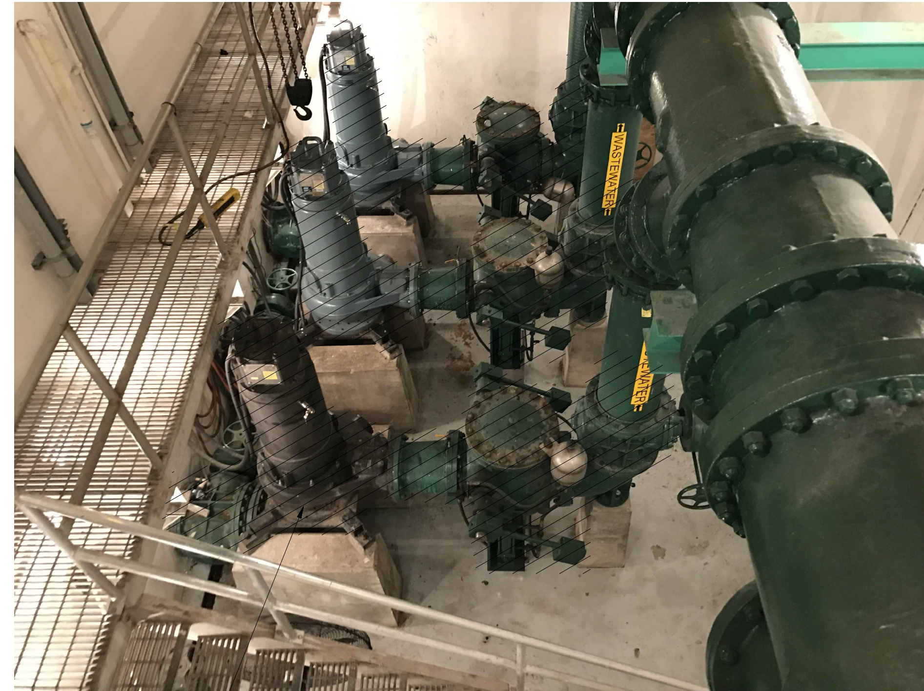
PUMP DEMOLITION NO SCALE
