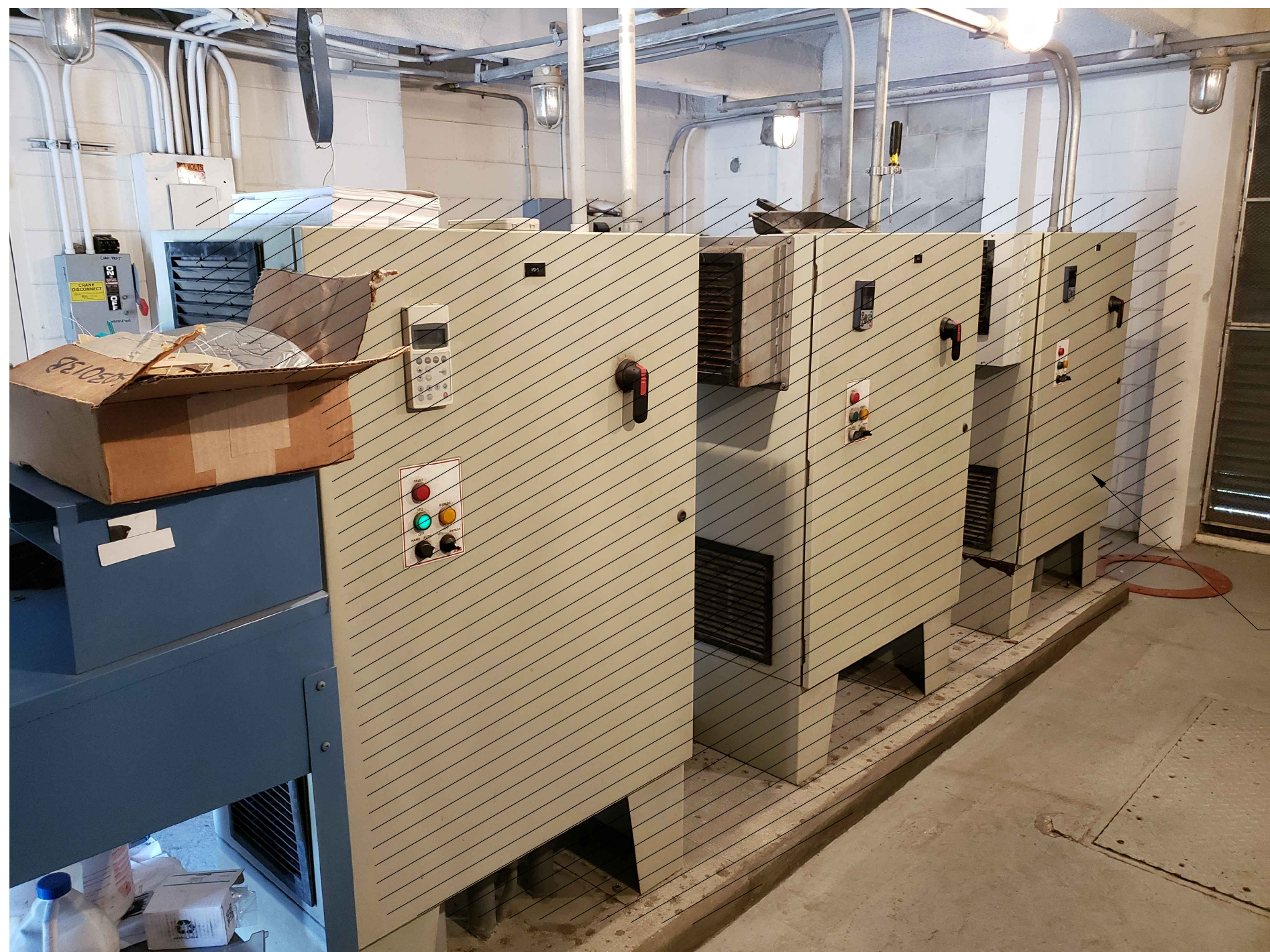
EXISTING AFD DEMOLITION NO SCALE
