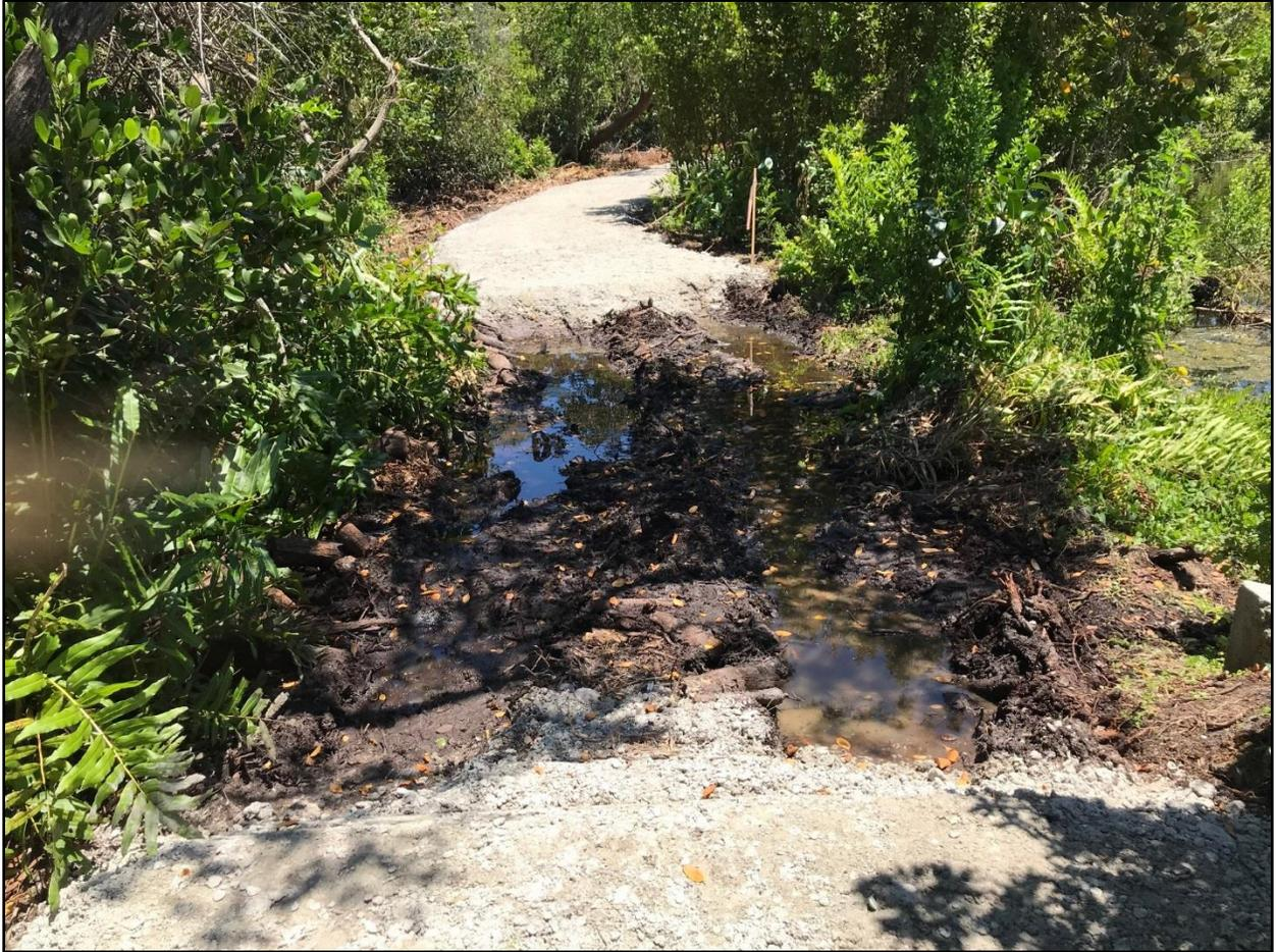
Site Photograph 2 - Boardwalk #3 location facing south. Boardwalk to connect existing shell trail areas to match grade on each side. This boardwalk shall be 25' long by 8' wide. Note this boardwalk shall include timbers that fully block views along its west face at a minimum of 8' tall from top of deck.
