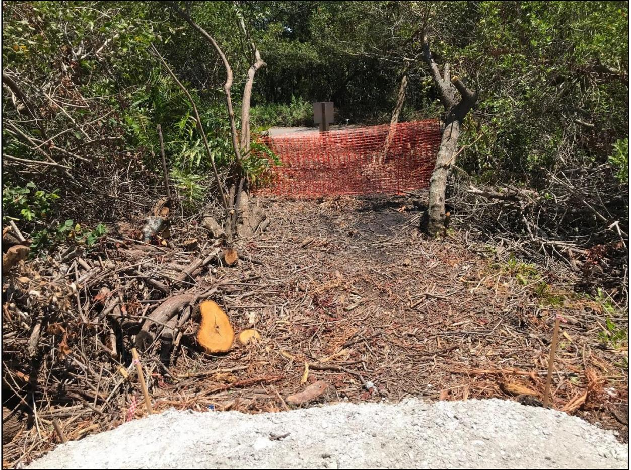
Site Photograph 3 - Boardwalk #4 location facing south. Boardwalk to connect existing shell trail areas to match grade on each side. This boardwalk shall be 48' long by 8' wide and tie in with an appropriate radius to the existing paved Trail at Robinson Preserve.
