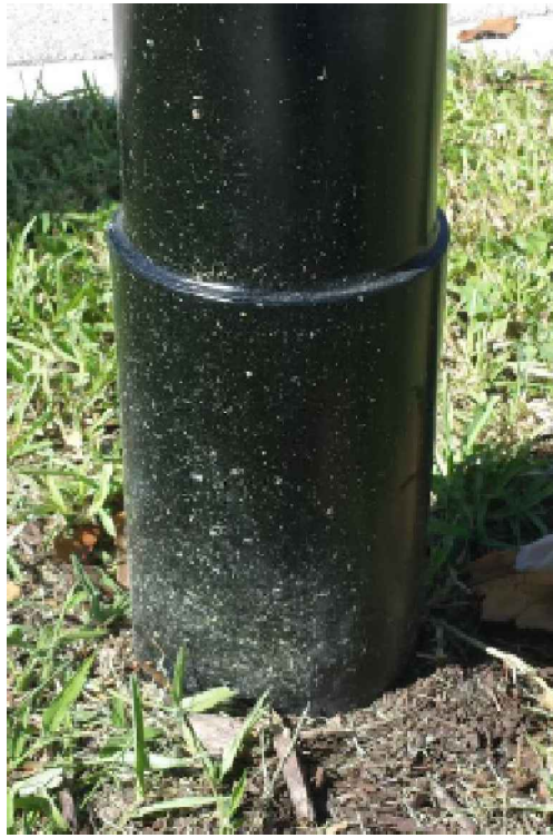
FIG.2 PROPER EMBEDMENT TO TAPE LINE
