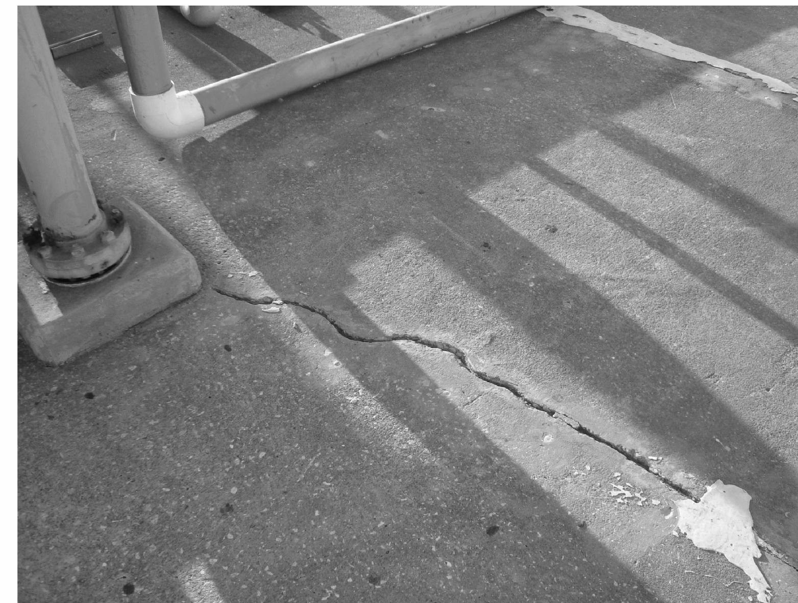
C REPAIR CRACKS IN CONCRETE
