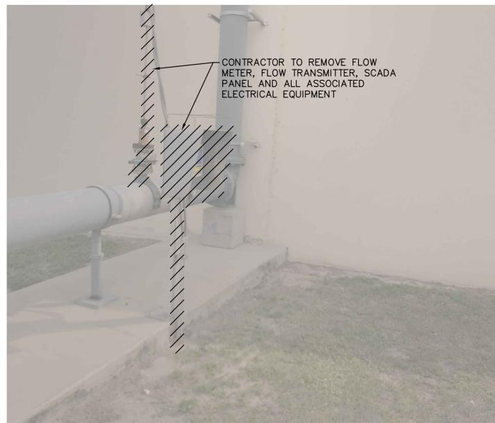
CONTRACTOR TO REMOVE FLOW METER, FLOW TRANSMITTER, SCADA PANEL AND ALL ASSOCIATED ELECTRICAL EQUIPMENT
