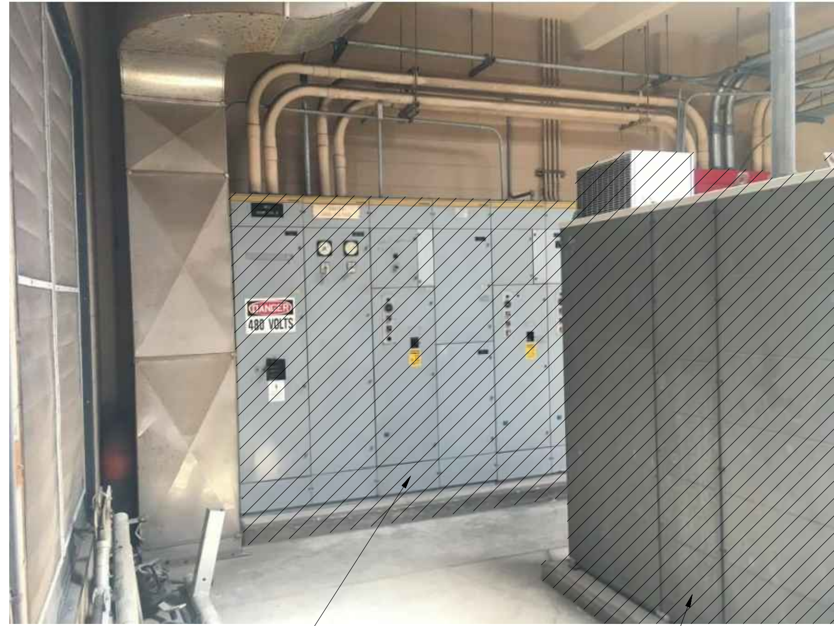
DEMOLISH EXISTING MCC PANELS AND HOUSEKEEPING PADS
