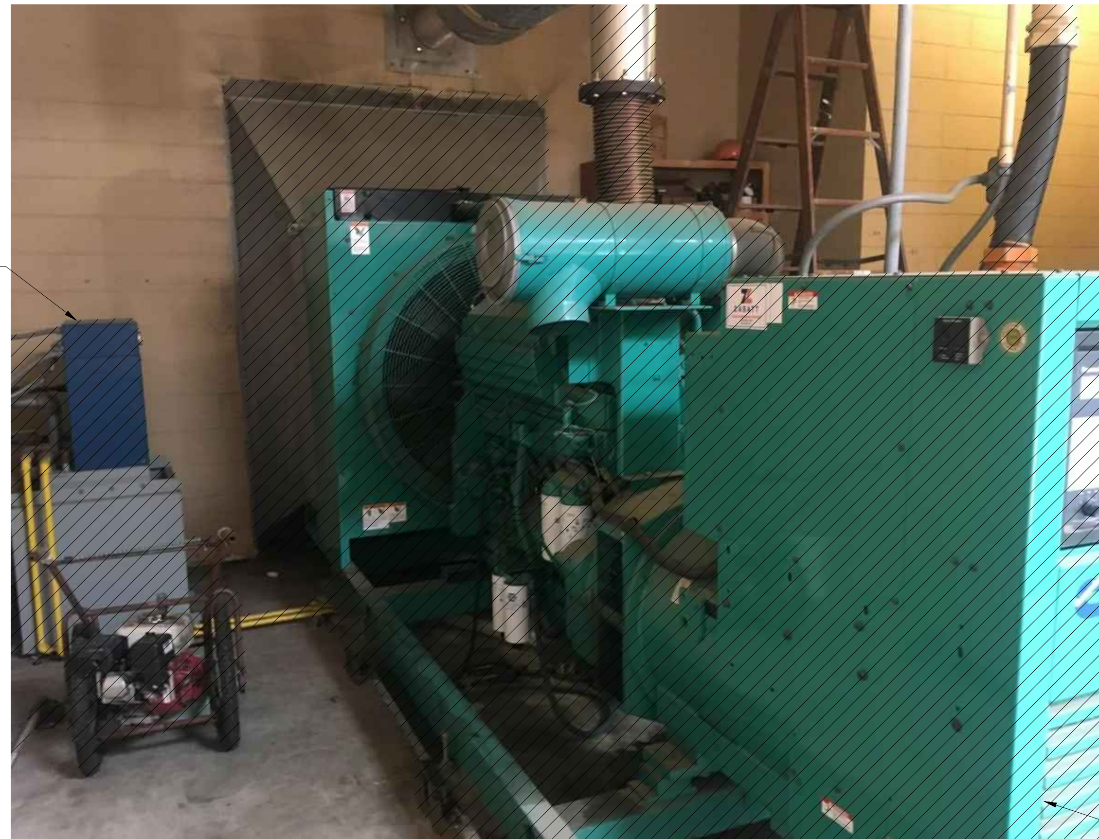
DEMOLISH FUEL DAY TANK AND FUEL PIPING
