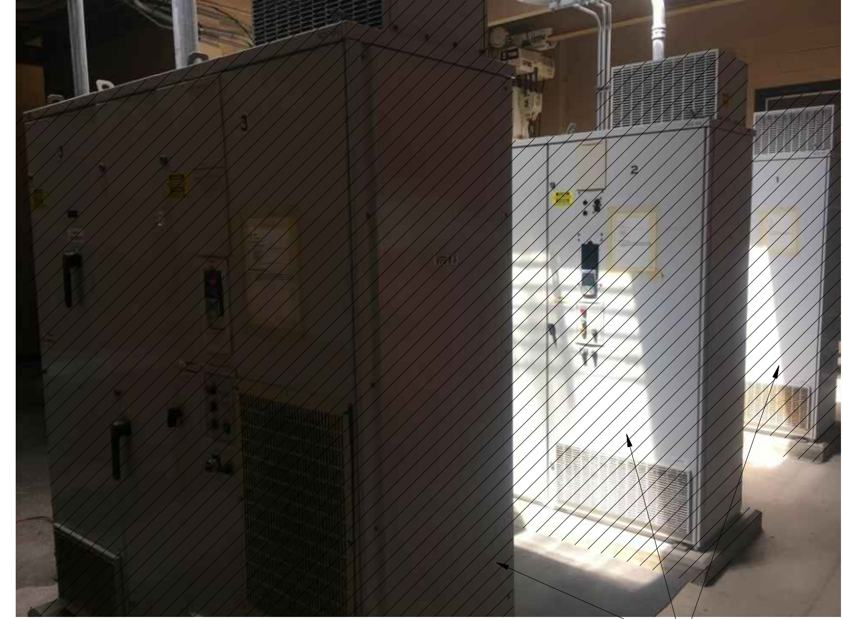
DEMOLISH EXISTING VFDS
