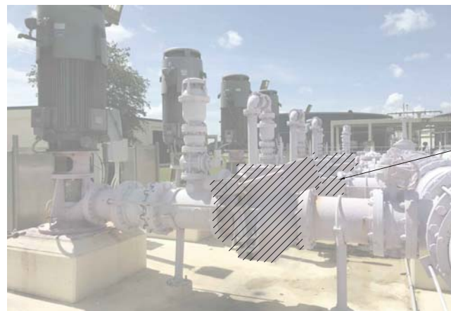
EX. 12" CHECK VALVE ASSEMBLY 4 N.T.S. CC-D-6
