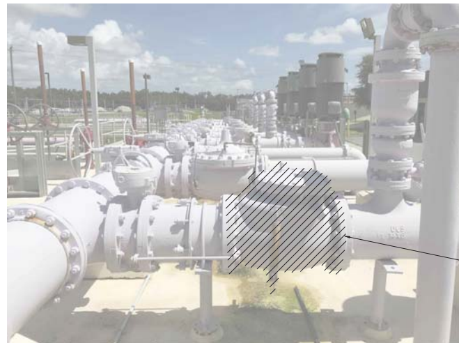
EX. 14" CHECK VALVE ASSEMBLY 2 N.T.S. CC-D-6
