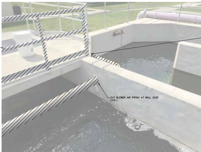
EX. SOUTH CCC BLOWER AIR PIPE PENETRATION 3 N.T.S. CC-D-4
