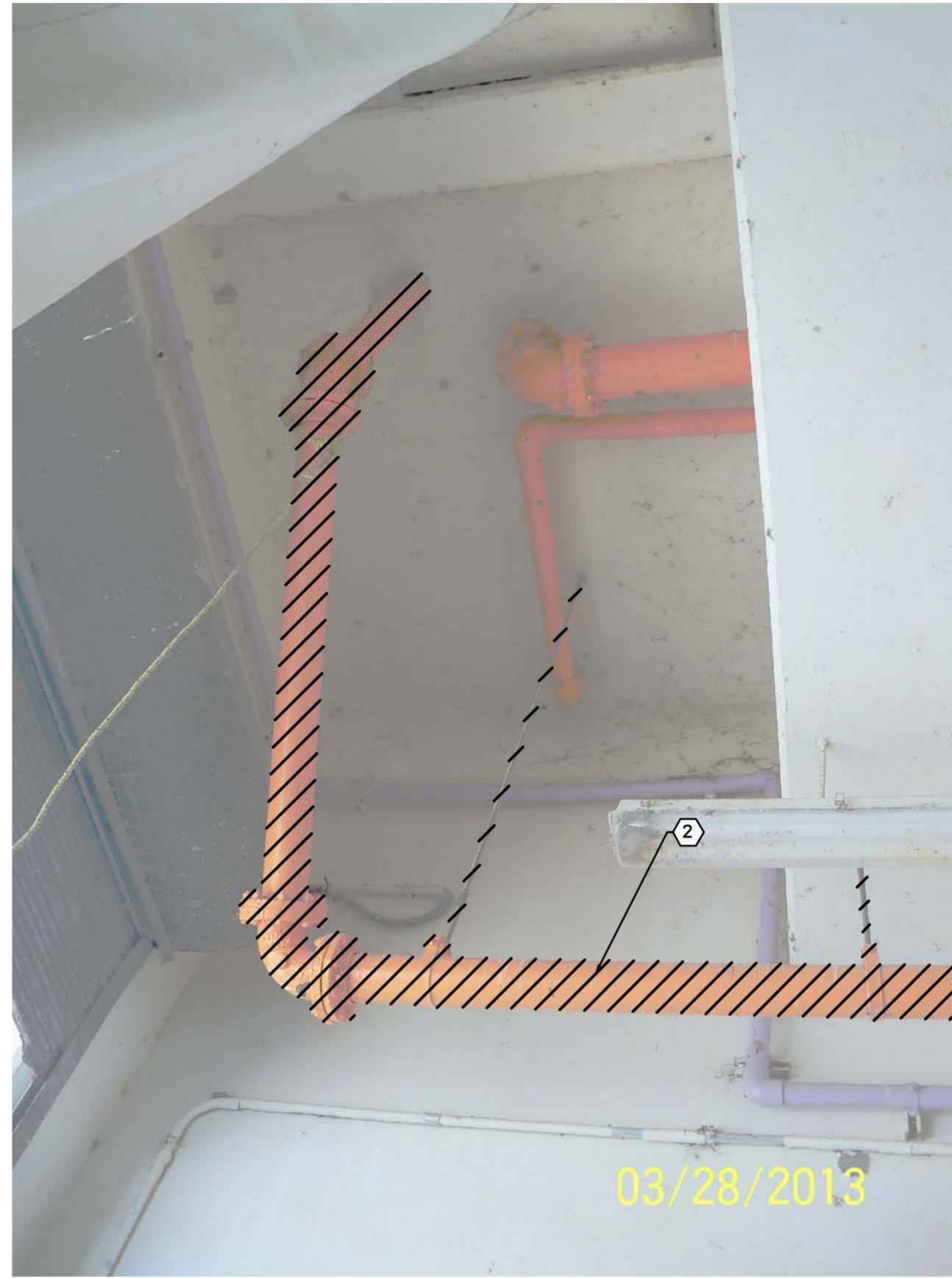
GRIT PIPE REMOVAL DETAIL 1 12 N.T.S. D-26
