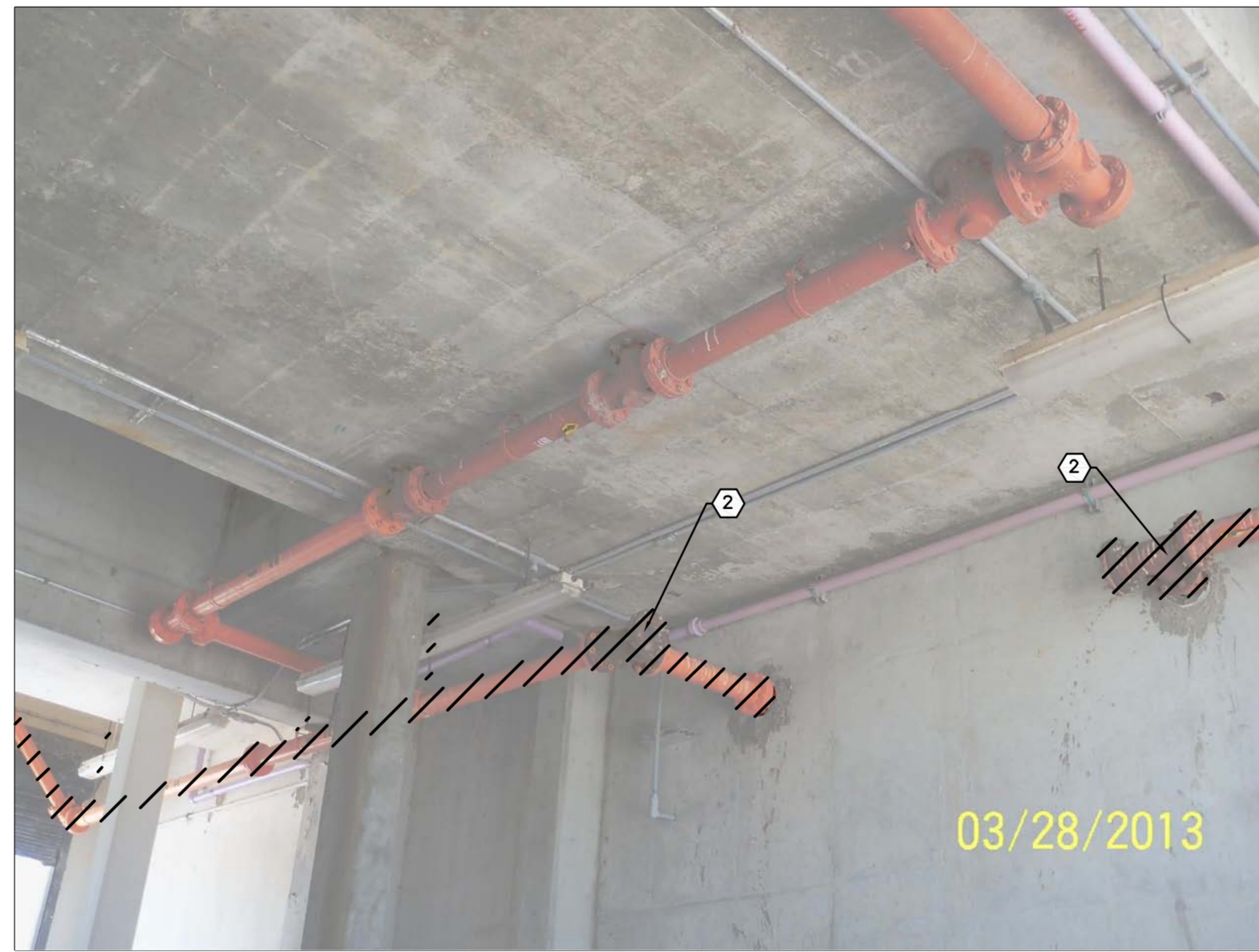
GRIT PIPE REMOVAL DETAIL 3 14 N.T.S. D-26
