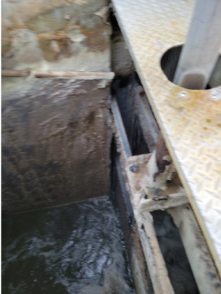
Figure 5: Corrosion at Stop Plate
