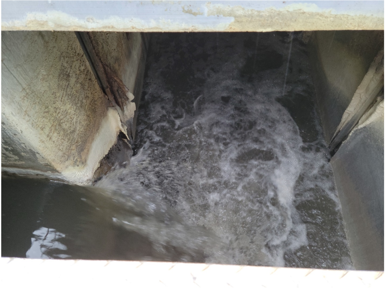
Figure 4: Corrosion at Stop Log Slots Downstream of Screen Channels
