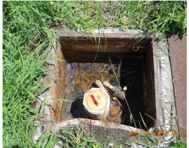
Site Photo 10: Product recovery well RW-3 with J-plug replacing original cap
