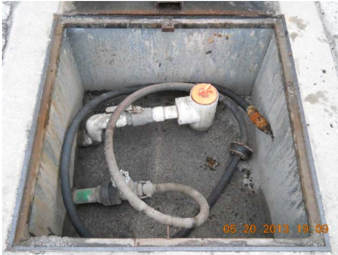
Site Photo 7: MPE well PRW-25 with Bellowsflex hose removed and new J-plug installed.
