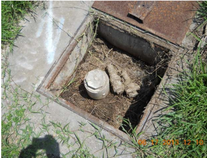
Site Photo 9: Product recovery well RW-4 with screw-on plastic well cap.
