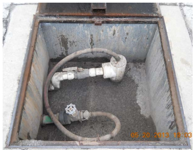
Site Photo 6: Example vault interior for MPE well components (PRW-25).
