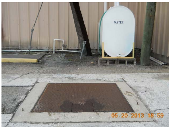
Photo 5: Example vault exterior for an MPE well (PRW-25).
