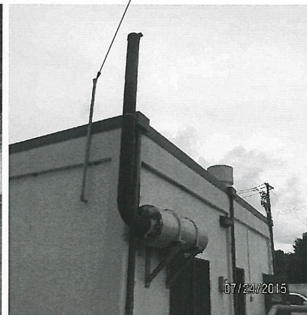
EXISTING GENERATOR MUFFLER - TO BE REMOVED (FACING SOUTH EAST)
