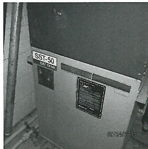
EXISTING DAY TANK (TANK, FUEL LINES, VENT, ETC.) (TO BE REMOVED)
