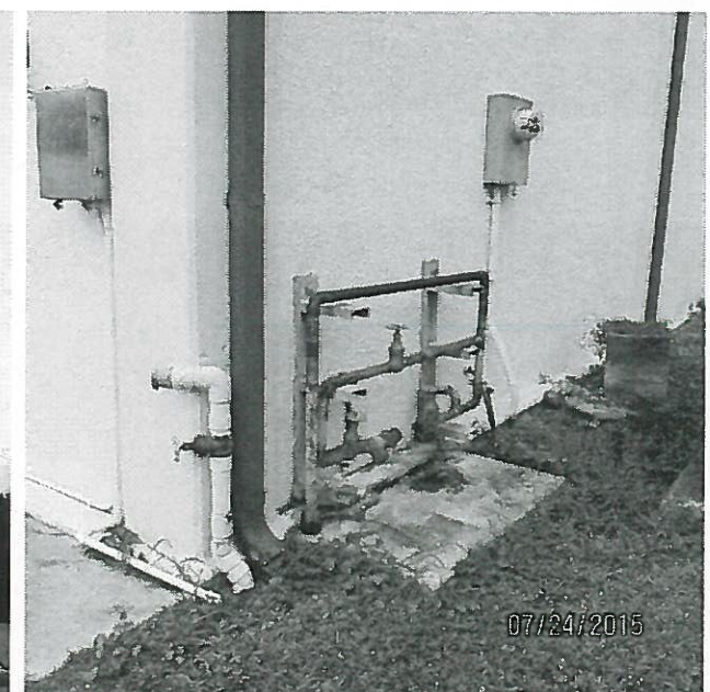
SITE PHOTO (FACING NORTH WEST)
